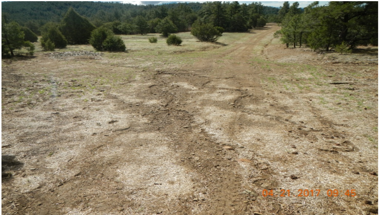
photo 3: There are minor signs of erosion at this area along the access road.
