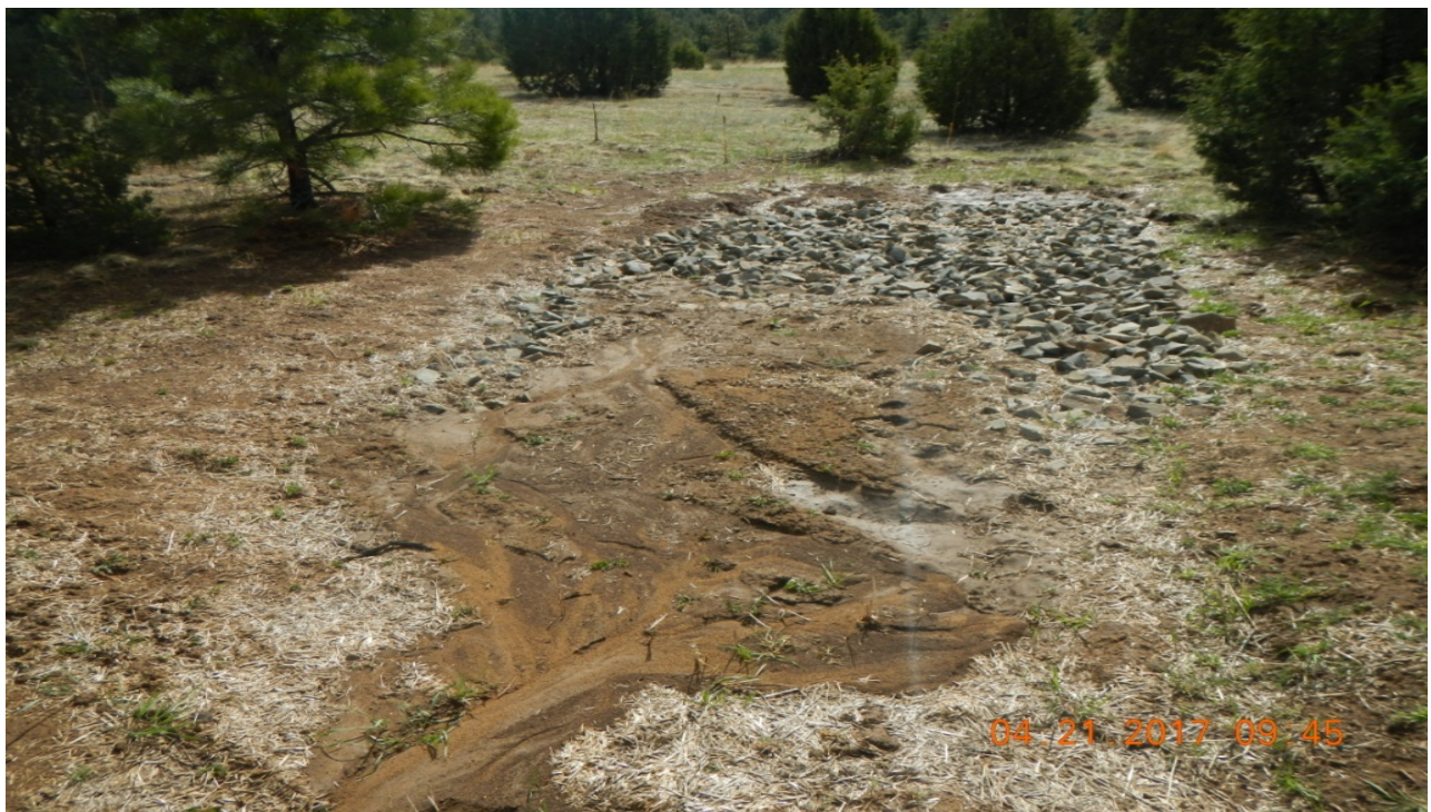
photo 4: Sediment is being deposited at the rock rip/rap.
