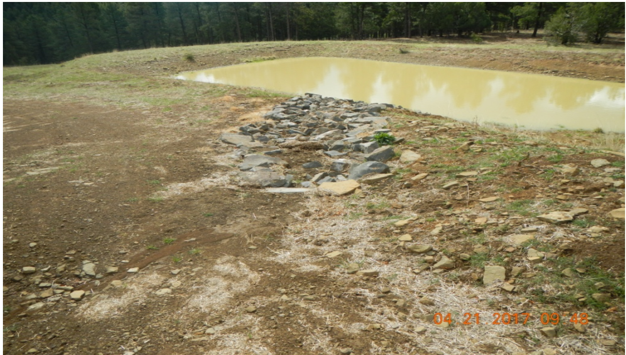
photo 7: Rock rip/rap is installed where stormwater is directed towards the pit.
