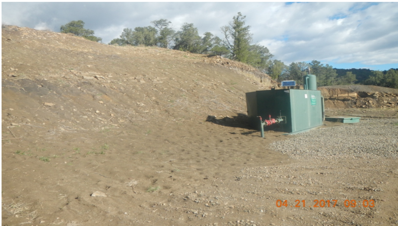
photo 2: Facing northwest toward the cut-slope. Sediment is being deposited around the equipment.
