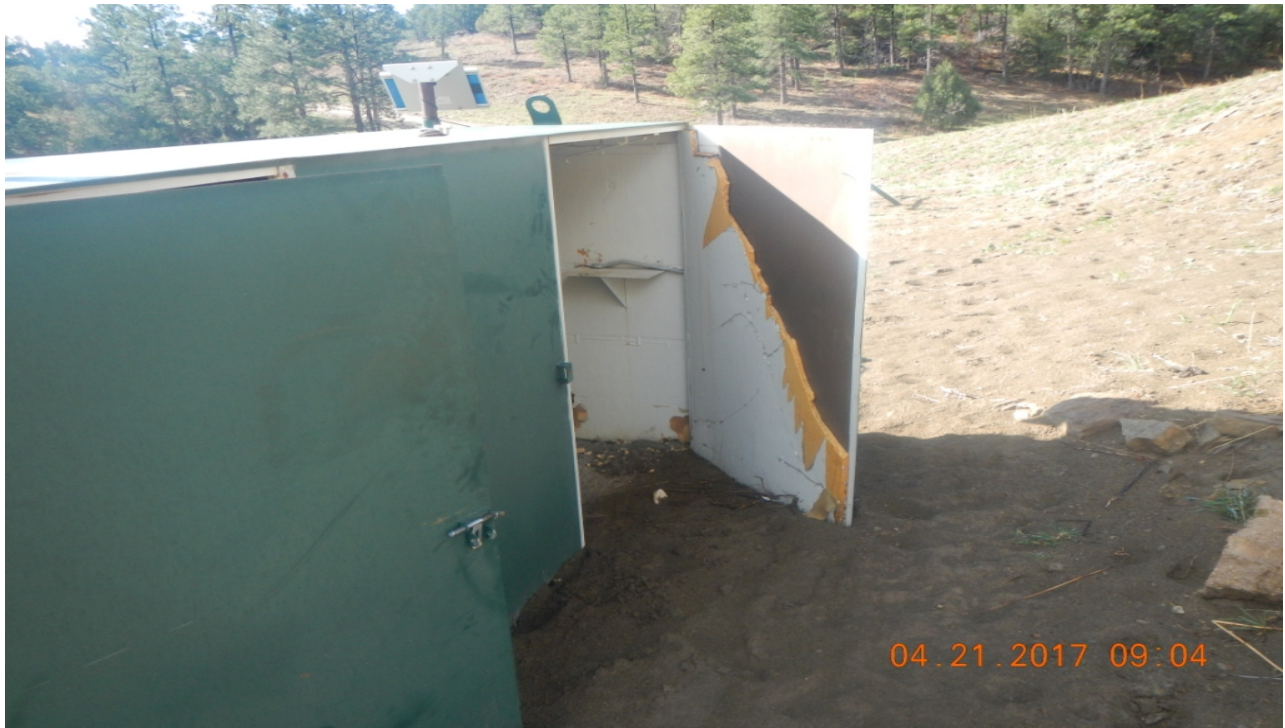
photo 3: The doors of this shed are open and sediment deposition prevents them from being closed.
