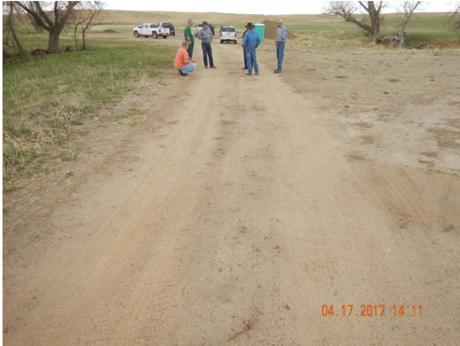
Photo 6: Photo taken from the access road east of the location, facing west. Surface owner had stated interest in leaving a portion of this road. A 502.b variance to not perform reclamation on portions of the road desired by the surface owner will need to be submitted and approved.
