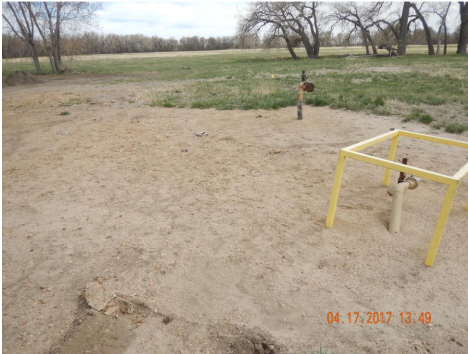
Photo 2: Photo taken from the west end of the location, facing south. Photo shows riser from flow/gathering system. Mr. Murphey from Lilis stated that Anadarko would be removing the lines on Wed. April 19 th
