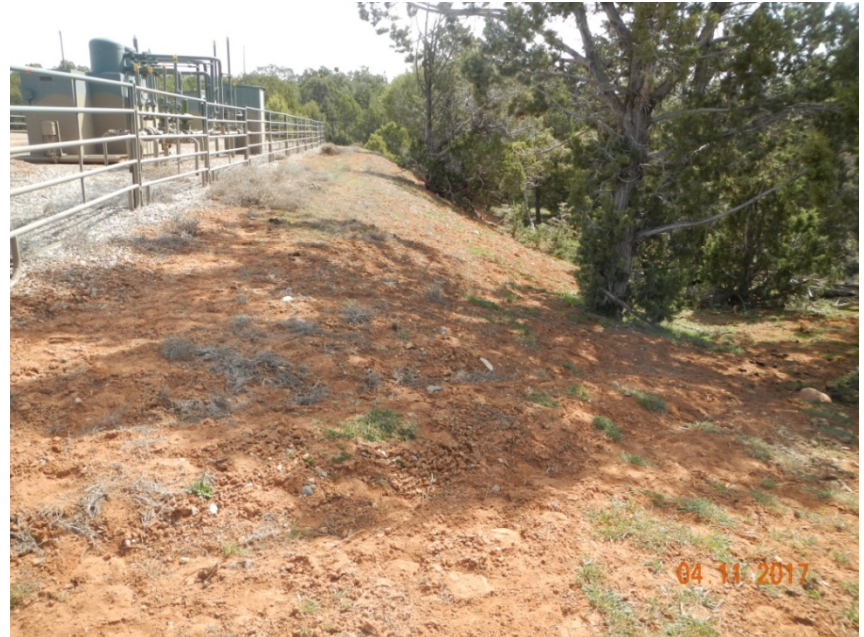
Photo 6: View of erosional channel approximately 1 foot wide and deep in the southwestern corner of the project area.
