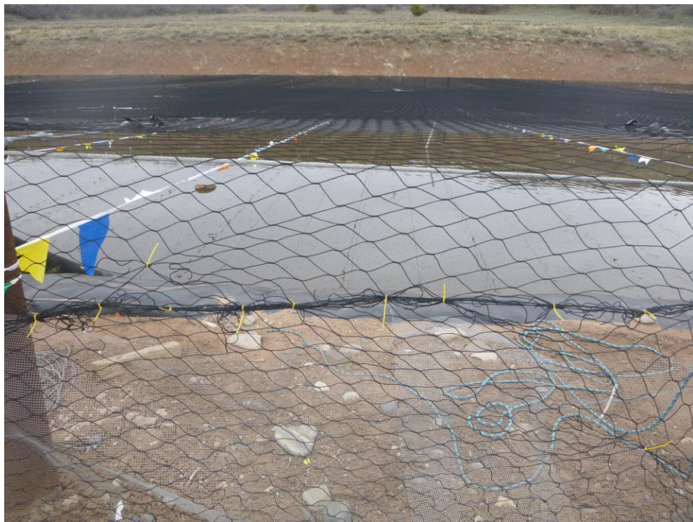
Photo 5: Damage to netting near manifold repaired.
