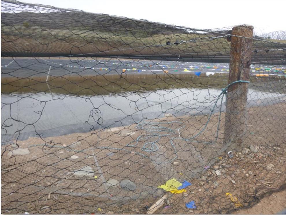
Photo 4: Damage to netting near manifold.
