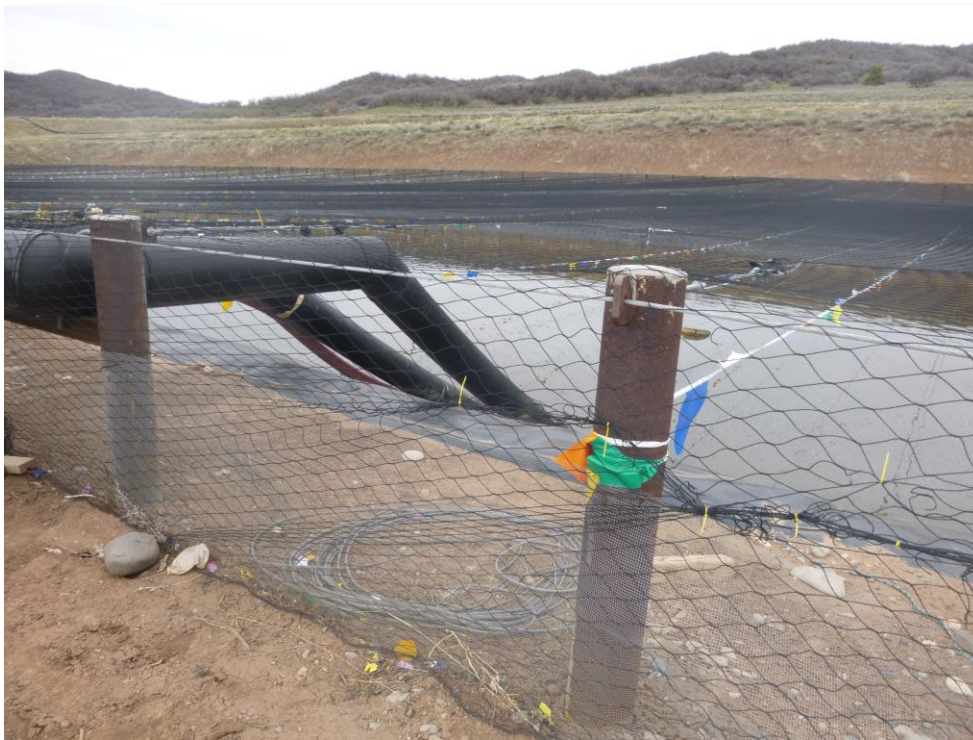
Photo 3: Damage to netting near manifold repaired.
