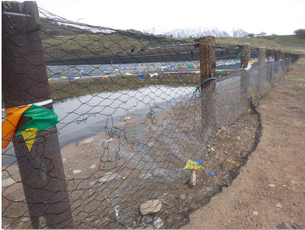
Photo 2: Damage to netting near manifold.
