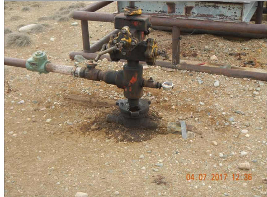
Photo 2. Stained soil at wellhead.
