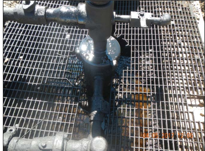
Photo 3. Cellar full of oily liquid without 2 feet of freeboard.
