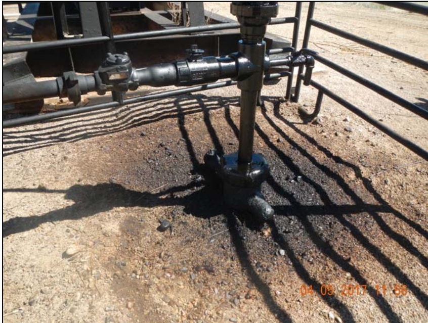
Photo 2. Ongoing leak at wellhead. Fresh oil and stained soil. 4/5/2017 Inspection
