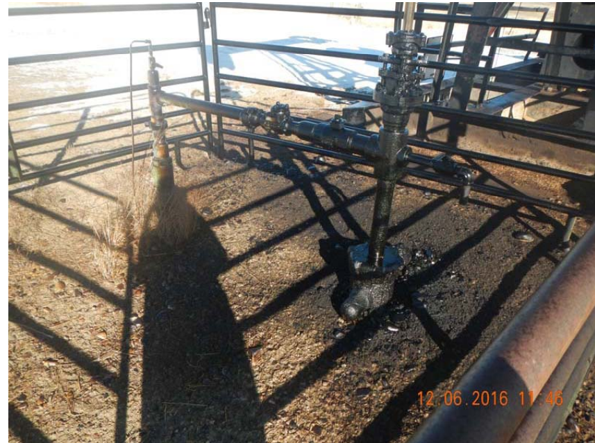
Photo 3. Ongoing leak at wellhead. Fresh oil and stained soil. 12/6/2016 Inspection
