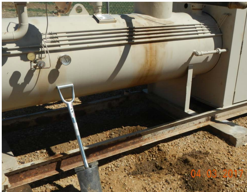
Stained soil under leaking pipe connection on separator.
