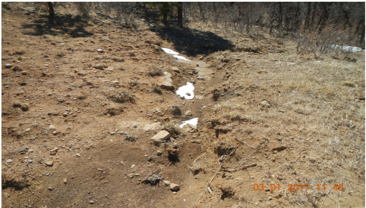
photo 6: There is an erosion channel off the south side of the location.
