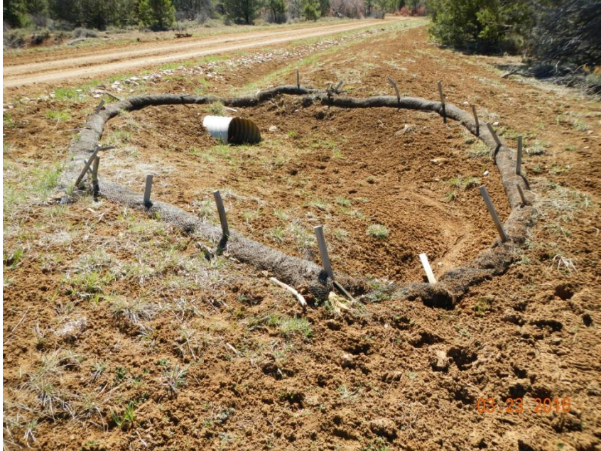
Photo 7: View of wattles along access road that are filling with sediment and need maintenance.
