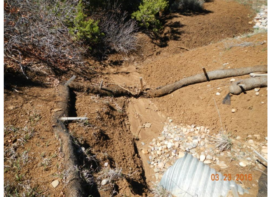
Photo 8: Another view of wattles along the access road that are filled with sediment and need maintenance or replacement.
