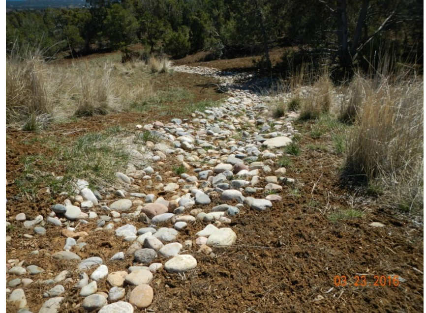
Photo 6: View of cobble run-down in the southern portion of the project area that appears to be functioning.
