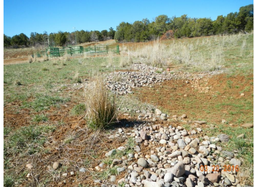
Photo 4: View of the northern portion of the project area from the northeastern edge facing westward. Cobble run-down appears to be functioning at this time.
