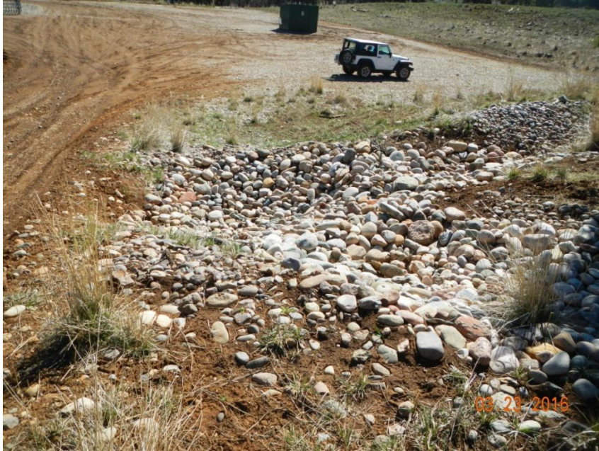
Photo 7: View of stormwater controls that appear to be functioning in the western portion of the project area.
