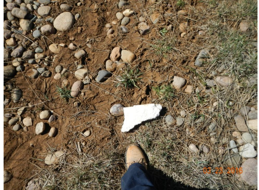
Photo 6: View of small styrofoam debris within the eastern interim reclamation area. Several small pieces of debris such as styrofoam, black liner material, etc. are scattered around the interim reclamation area and need to be removed and properly disposed of.
