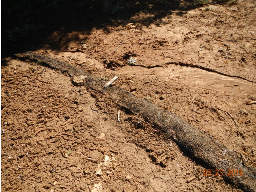
Photo 9: View of wattles in the eastern portion of the project area that are no longer functioning.
