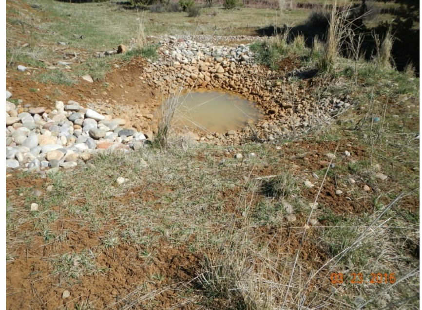
Photo 8: View of silt trap in the southeastern portion of the project area that appears to be functioning.
