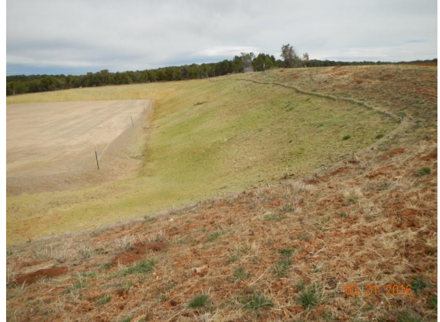
Photo 2: View of eastern portion of the project area from the southeastern corner facing northward. Cut and fill slopes have been seeded and/or tackified with mulch applied. Revegetation is occurring in portions of the outer disturbance areas with wheatgrasses and sandberg bluegrass ( Poa secunda ).
