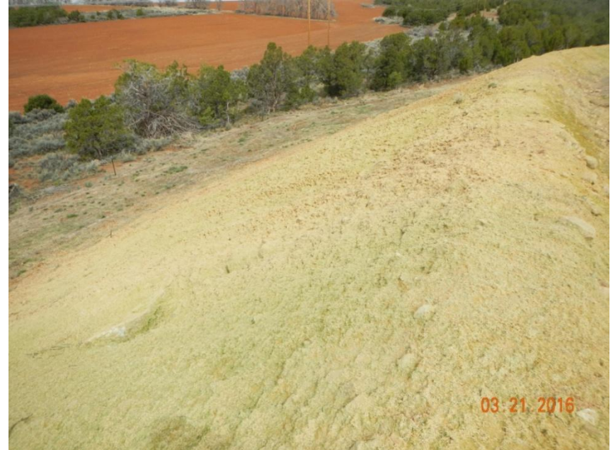
Photo 4: View of the western portion of the project area from the southwestern corner facing northward. Light green is tackifier and mulch on slope.
