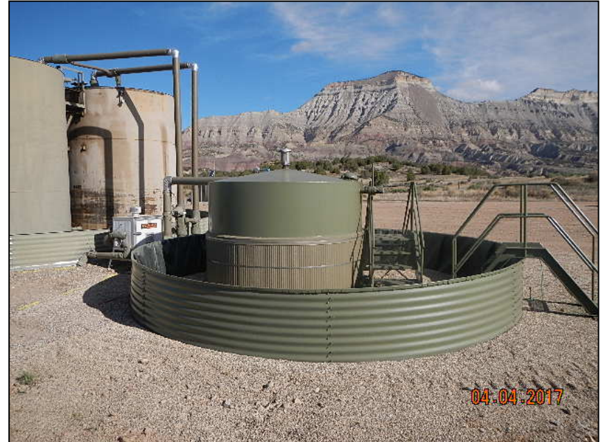
Photo 2. Tank missing signage.
