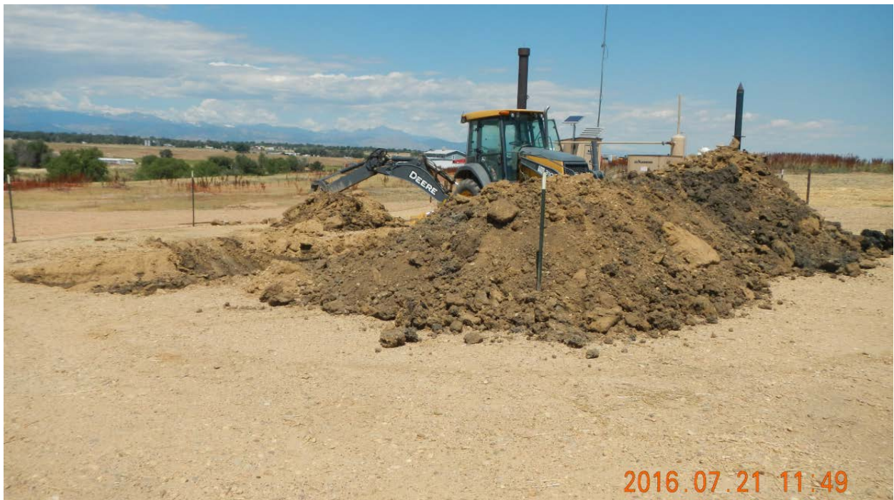
Spoils bank created by excavation to expose dump line
