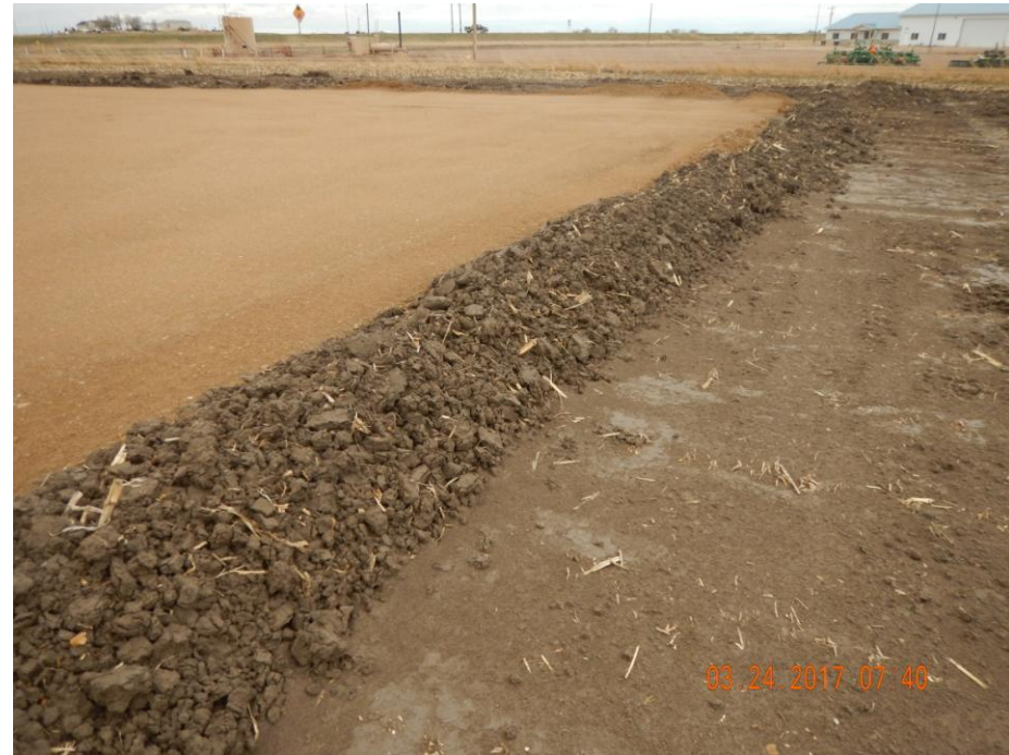
Photo 7: Photo taken from the north end of the location, facing west. Photo shows berm on the north end has not been consolidated and not in proper functioning condition. Without proper consolidation berms along the location perimeter will increase the sediment laden stormwater runoff from the location.
