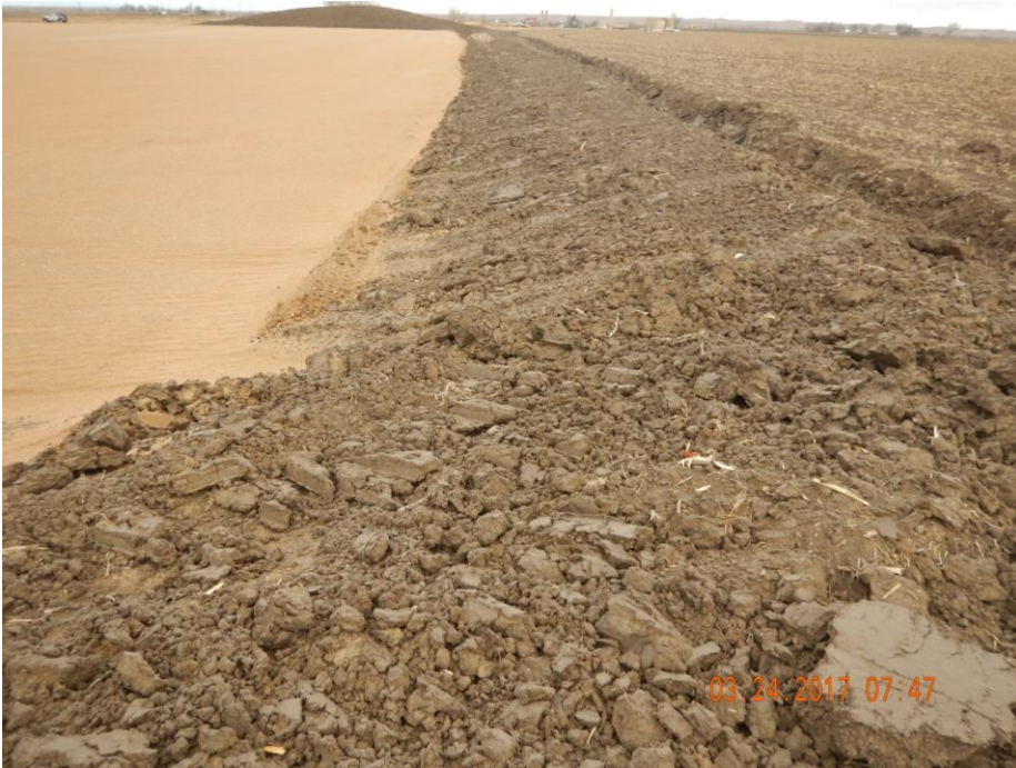
Photo 19: Photo taken from the south east end of the location, facing north. Photo shows slopes on the eastern perimeter of the location have been insufficiently consolidated and improperly tracked.
