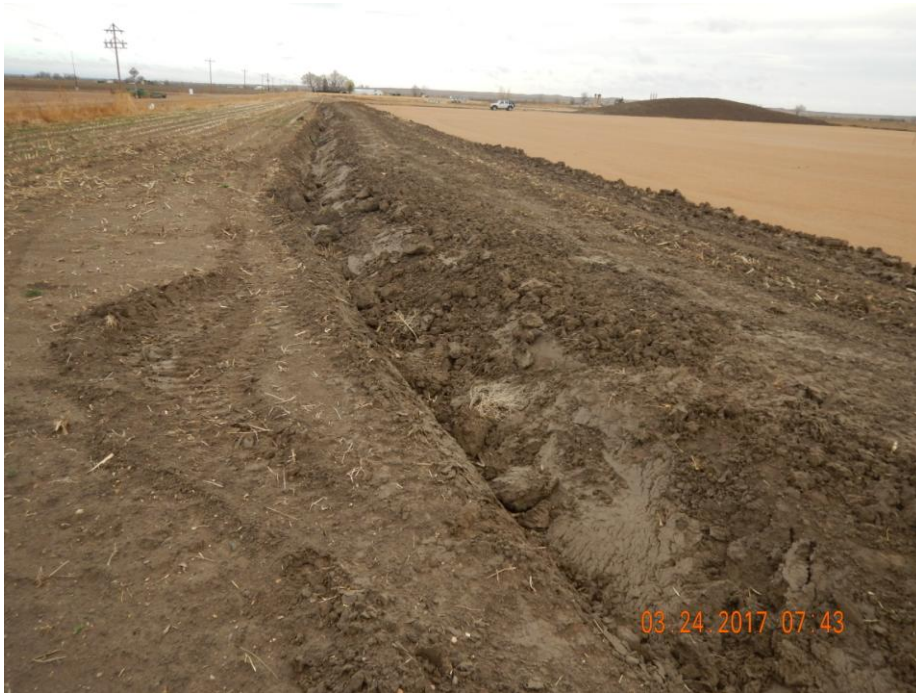
Photo 13: Photo taken from the southwest corner of the location, facing north. Photo shows stormwater ditch; Stormwater ditch has not been consolidated. Without proper consolidation this ditch will increase the sediment laden stormwater runoff from the location.
