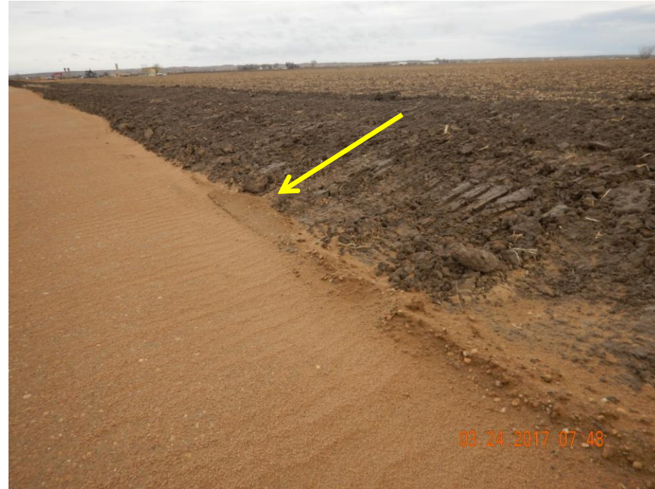
Photo 20: Photo taken from the east end of the location, facing northeast. Photo shows slopes on the eastern perimeter of the location have been improperly tracked. Yellow arrow shows direction of slope. Tracking should be perpendicular to the slope in order to reduce runoff velocity and erosion.
