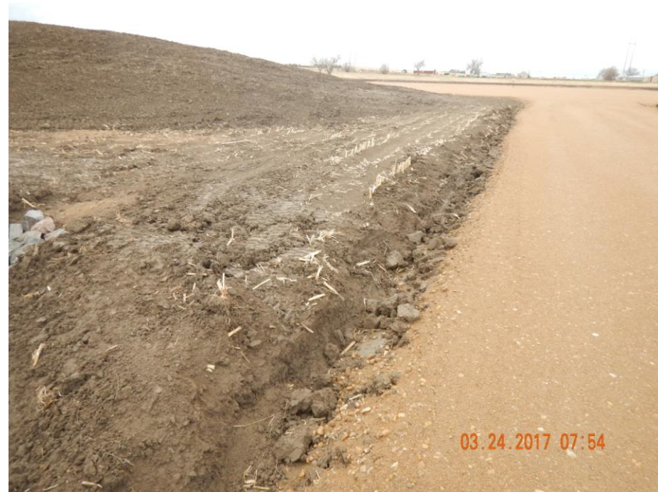
Photo 32: Photo taken from the north end of the location, facing south. Photo shows stormwater ditch has not been consolidated. Without proper consolidation this ditch will increase the sediment laden stormwater runoff from the location.
