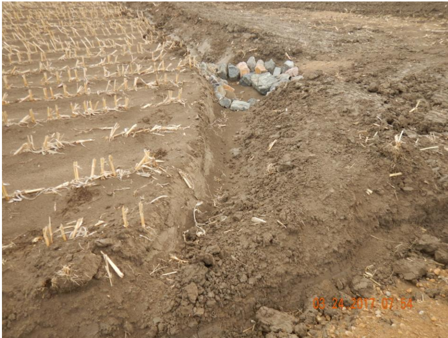
Photo 31: Photo taken from the north end of the location (east of access road). Photo shows sediment trap BMP. BMP has filled with sediment and will require maintenance.
