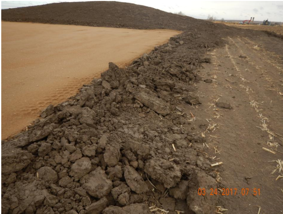
Photo 25: Photo taken from the east end of the location, facing north. Photo shows berm has not been consolidated and not in proper functioning condition. Without proper consolidation berms along the location perimeter will increase sediment laden stormwater runoff from the location.
