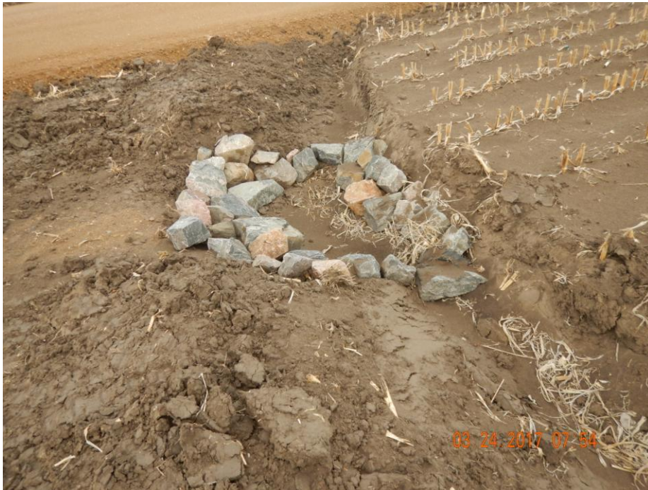
Photo 29: Photo taken from the north end of the location (east of access road). Photo shows sediment trap BMP. BMP has filled with sediment and will require maintenance. It appears only large-sized rock aggregate have been utilized to construct the BMP; using only large aggregates can contribute to erosion degradation as stormwater can be accelerated around or under the material, expanding stormwater impacts and rendering the BMP inadequate. This is becoming evident in areas shown by the yellow arrows
