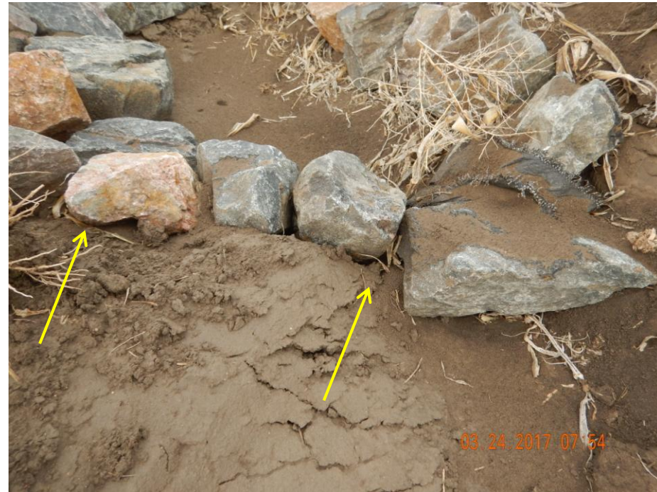
Photo 30: Photo taken from the north end of the location (east of access road). Photo shows sediment trap BMP. BMP has filled with sediment and will require maintenance. It appears only large-sized rock aggregate have been utilized to construct the BMP; using only large aggregates can contribute to erosion degradation as stormwater can be accelerated around or under the material, expanding stormwater impacts and rendering the BMP inadequate. This is becoming evident in areas shown by the yellow arrows
