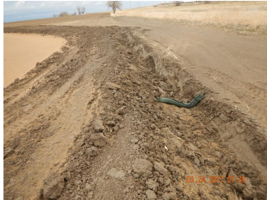
Photo 16: Photo taken from the north end of the location. Photo shows stormwater ditch has not been consolidated. Without proper consolidation this ditch will increase the sediment laden stormwater runoff from the location. Photo also shows wattle used as a stormwater and sediment control BMP. Wattle BMP has not been properly installed by trenching and backfilling the wattle.
