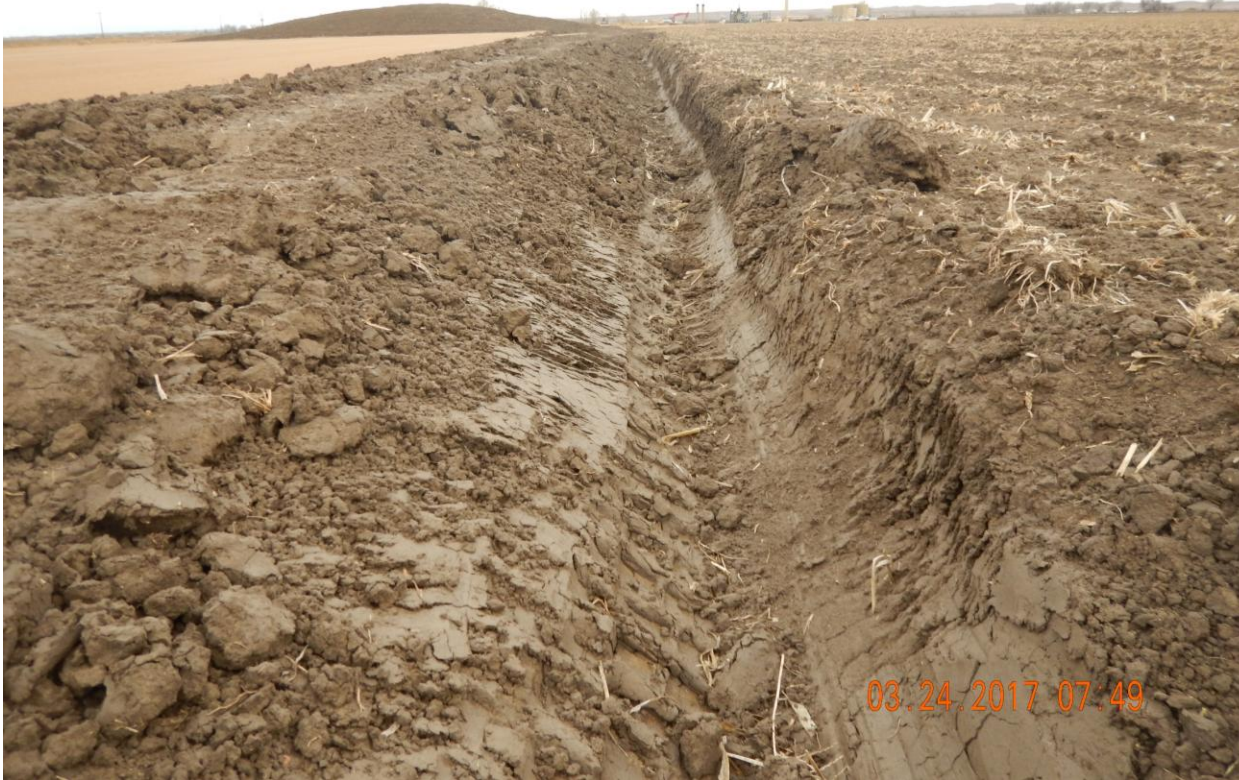
Photo 22: Photo taken from the stormwater ditch on the east end of the location. Photo shows stormwater ditch has not been consolidated and has been constructed with a steep grade. Without proper consolidation and grade, ditch will increase the sediment laden stormwater runoff from the location. CDOT recommends ditches be constructed with a grade of 2:1.
