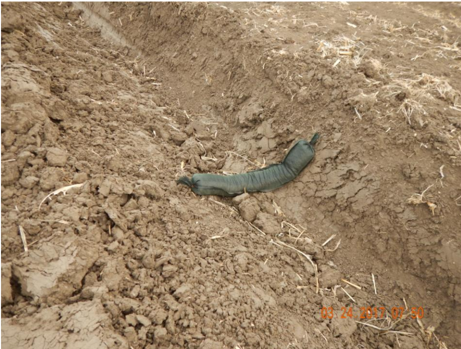
Photo 23: Photo taken from the east end of the location. Photo shows wattle used as a stormwater and sediment control BMP. Wattle BMP has not been properly installed by trenching and backfilling the wattle, and is not in proper functioning condition.
