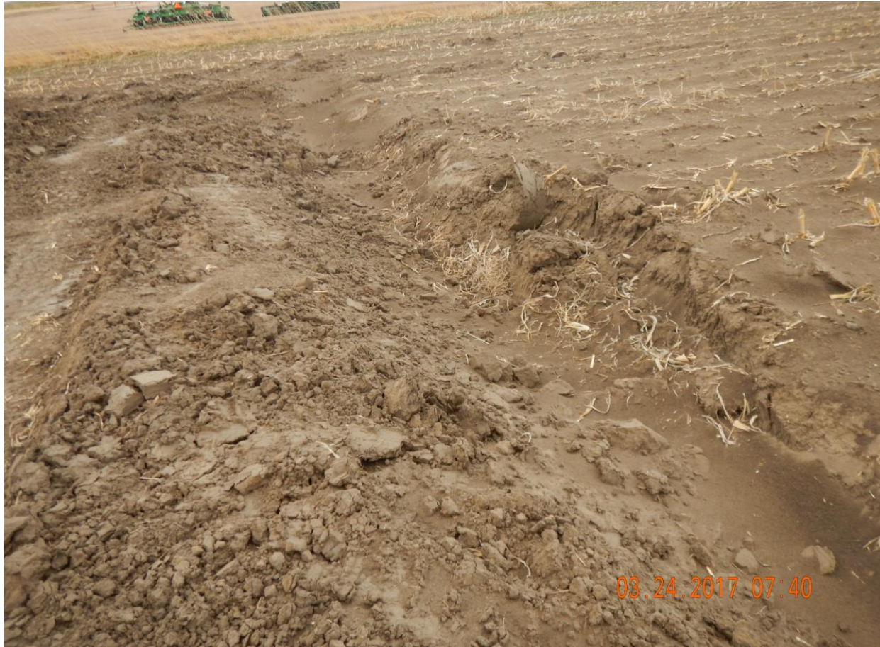
Photo 8: Photo taken from the north end of the location. Photo shows stormwater ditch has filled with sediment and will require maintenance. Stormwater ditch has not been consolidated. Without proper consolidation this ditch will increase the sediment laden stormwater runoff from the location.
