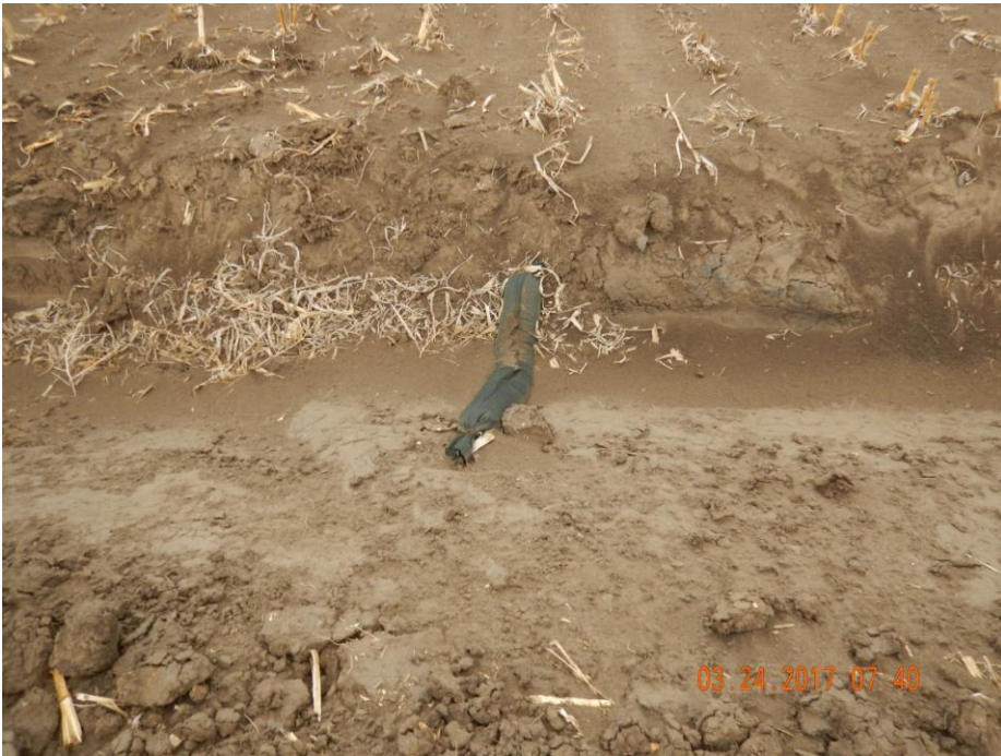
Photo 6: Photo taken from the stormwater control ditch on the north end of the location. Photo shows wattle BMP has filled with sediment and will require maintenance.
