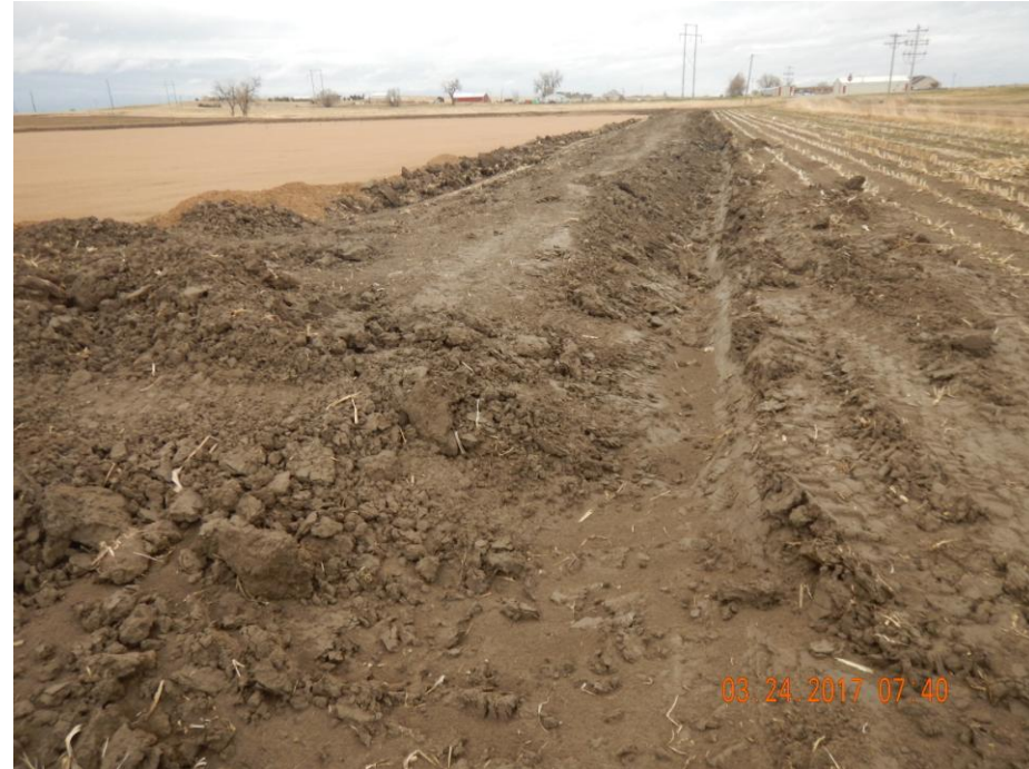
Photo 10: Photo taken from the northwest corner of the location, facing south. Photo shows stormwater ditch; Stormwater ditch has not been consolidated. Without proper consolidation this ditch will increase the sediment laden stormwater runoff from the location.
