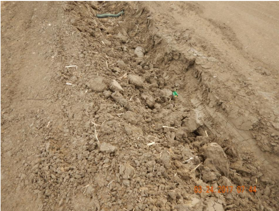
Photo 15: Photo taken from the north end of the location. Photo shows stormwater ditch has not been consolidated. Without proper consolidation this ditch will increase the sediment laden stormwater runoff from the location.
