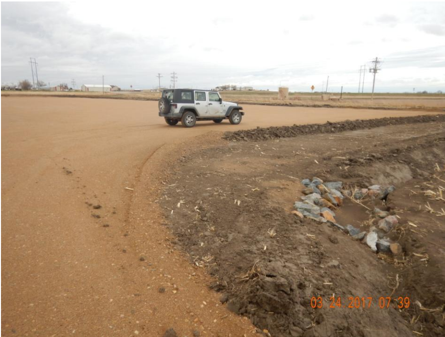
Photo 3: Photo taken from the north end of the location facing southwest. Photo shows pad has largely been stabilized with initial pad construction activities appearing to have been completed.
