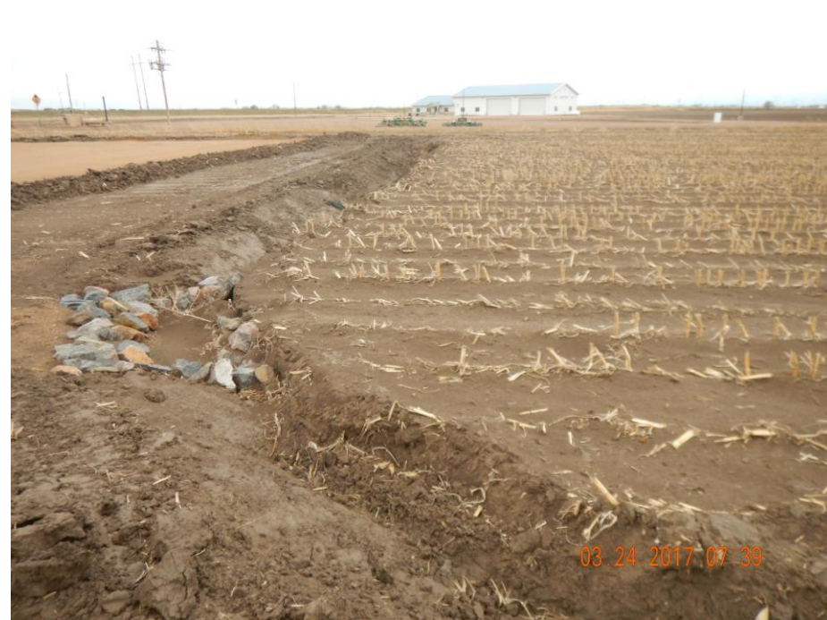
Photo 4: Photo taken from the north end of the location facing west. Photo shows perimeter stormwater control ditch and rock sediment trap BMPs
