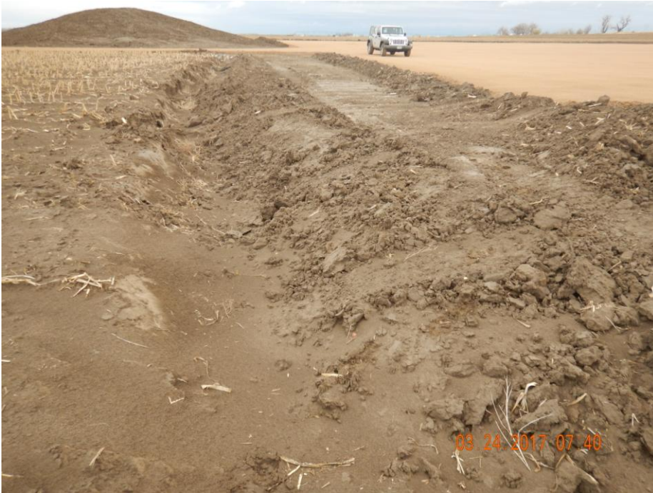
Photo 9: Photo taken from the northwest corner of the location, facing east. Photo shows stormwater ditch has filled with sediment and will require maintenance. Stormwater ditch has not been consolidated. Without proper consolidation this ditch will increase the sediment laden stormwater runoff from the location.
