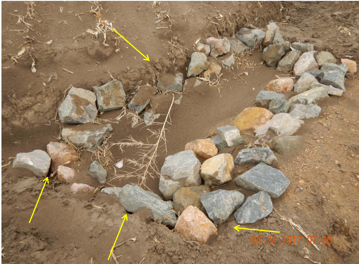
Photo 5: Photo taken from the northwest end of the location. Photo shows sediment trap BMP. BMP has filled with sediment and will require maintenance. It appears only large-sized rock aggregate have been utilized to construct the BMP; using only large aggregates can contribute to erosion degradation as stormwater can be accelerated around or under the material, expanding stormwater impacts and rendering the BMP inadequate. This is becoming evident in areas shown by the yellow arrows
