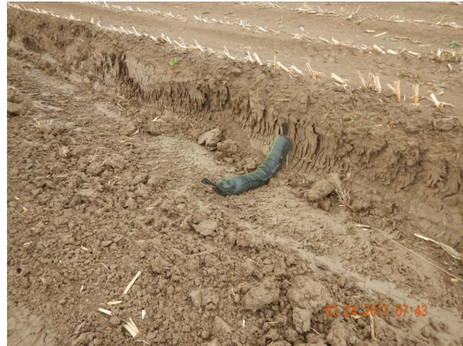
Photo 12: Photo taken from the west end of the location. Photo shows wattle used as a stormwater and sediment control BMP. Wattle BMP has not been properly installed by trenching and backfilling the wattle. Photo also shows stormwater ditch has not been consolidated and has been constructed with a steep grade. Without proper consolidation and grade this ditch will increase the sediment laden stormwater runoff from the location. CDOT recommends ditches be constructed with a grade of 2:1.
