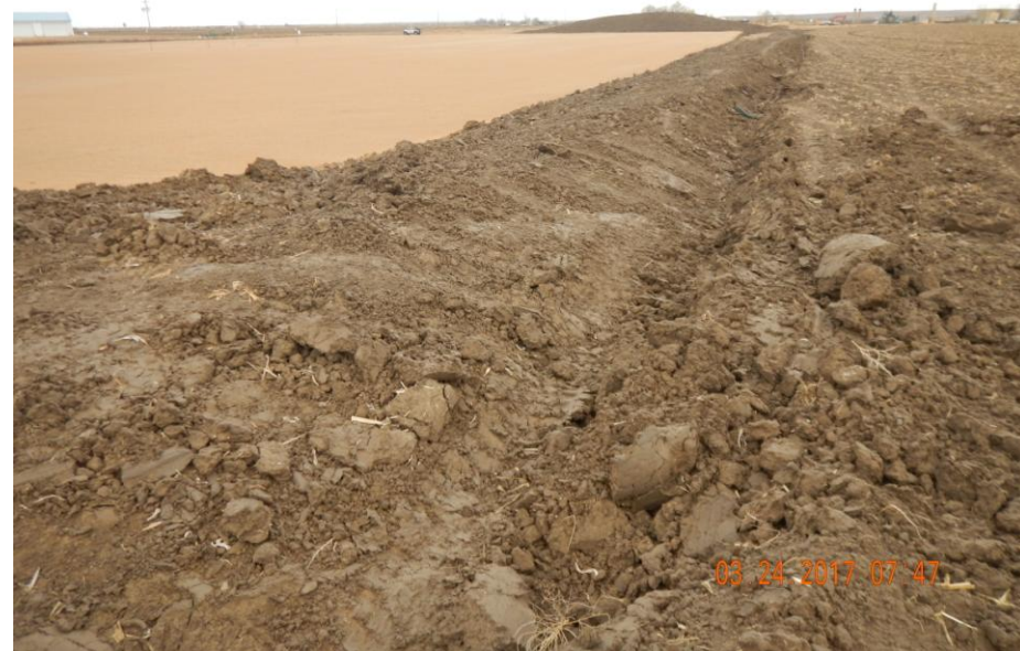
Photo 18: Photo taken from the southeast corner of the location, facing north. Photo shows stormwater ditch; Stormwater ditch has not been consolidated. Without proper consolidation this ditch will increase the sediment laden stormwater runoff from the location.
