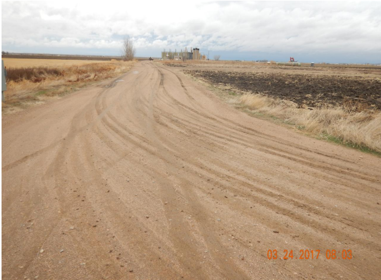
Photo 33: Photo taken from the intersection of CR 63 and the access road. Access road leads to three separate locations operated by BBC. Photo shows no vehicle tracking BMPs has been implemented to mitigate sediment tracked from the construction site, or the locations, onto roadways.
