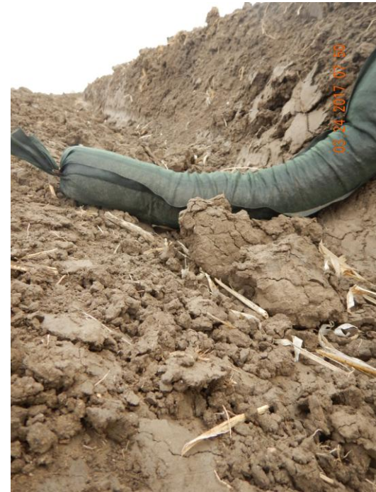
Photo 24: Photo taken from the east end of the location. Photo shows wattle used as a stormwater and sediment control BMP. Wattle BMP has not been properly installed by trenching and backfilling the wattle, and is not in proper functioning condition. Photo also shows stormwater ditch has been constructed with a steep grade. CDOT recommends ditches be constructed with a grade of 2:1.
