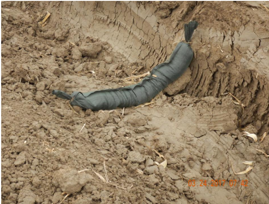
Photo 11: Photo taken from the west end of the location. Photo shows wattle used as a stormwater and sediment control BMP. Wattle BMP has not been properly installed by trenching and backfilling the wattle.
