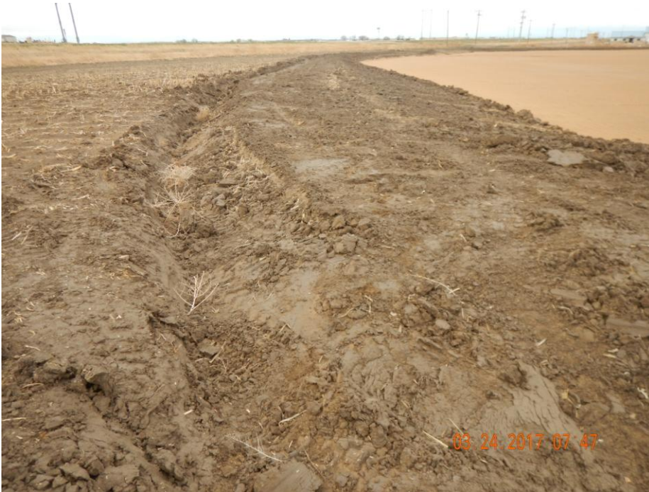
Photo 17: Photo taken from the southeast corner of the location, facing west. Photo shows stormwater ditch; Stormwater ditch has not been consolidated. Without proper consolidation this ditch will increase the sediment laden stormwater runoff from the location.
