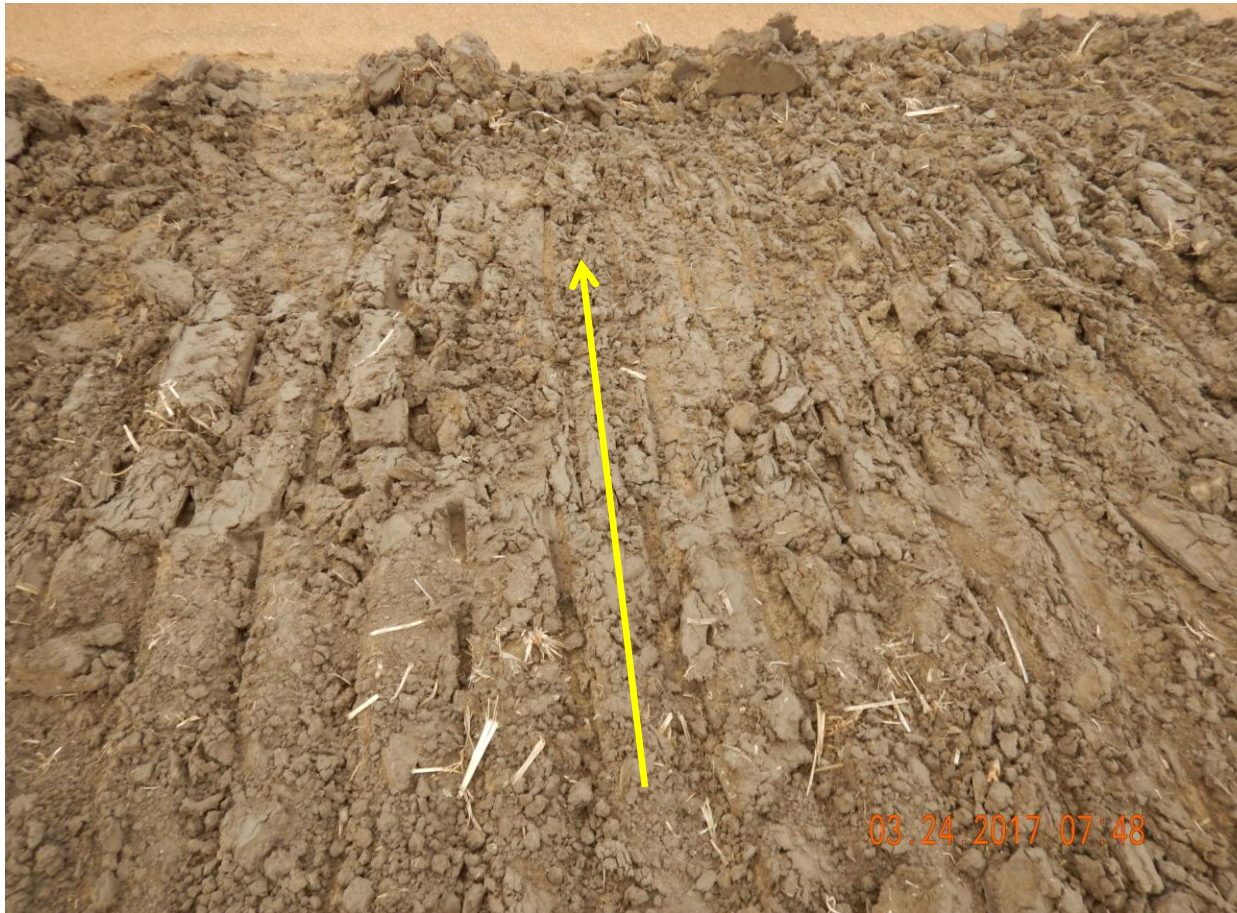
Photo 21: Photo taken from the east end of the location. Photo shows slopes on the eastern perimeter of the location have been improperly tracked. Yellow arrow shows direction of slope. Tracking should be perpendicular to the slope in order to reduce runoff velocity and erosion.
