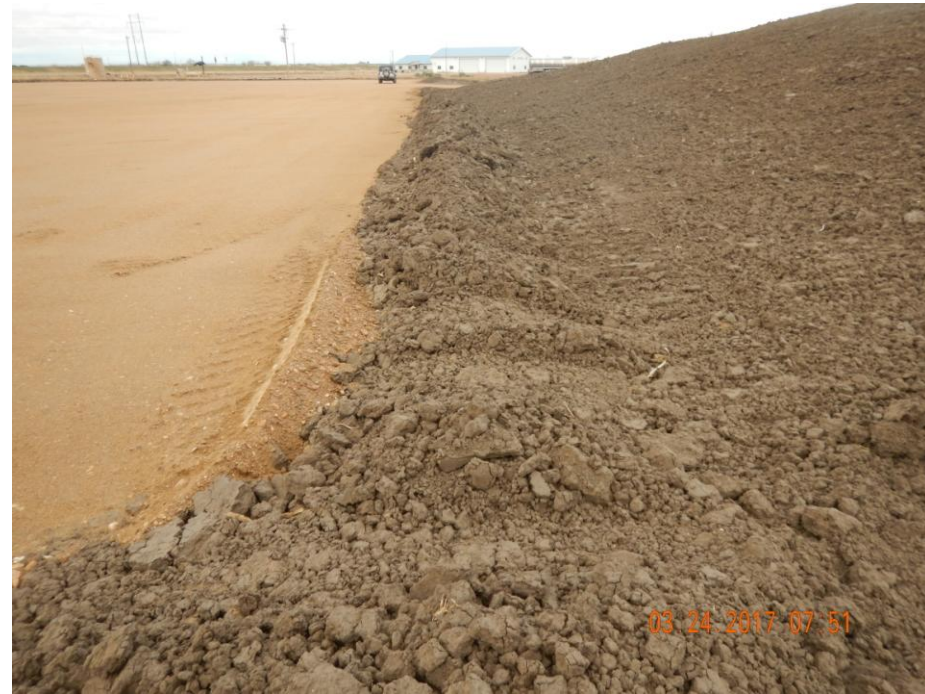
Photo 26: Photo taken from the southeast end of the topsoil pile. Photo shows berm has not been consolidated. Without proper consolidation berms along the location perimeter will increase sediment laden stormwater runoff from the location.
