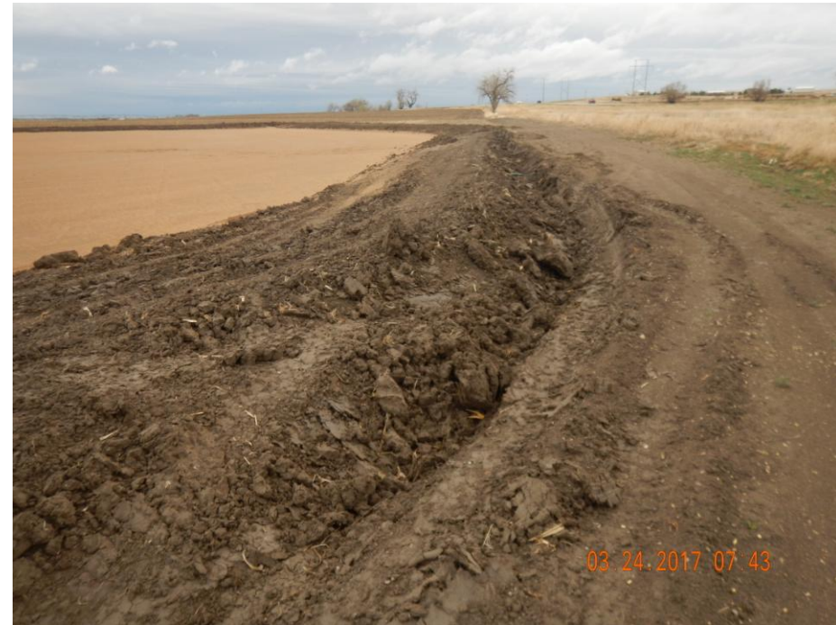
Photo 14: Photo taken from the southwest corner of the location, facing north. Photo shows stormwater ditch; Stormwater ditch has not been consolidated. Without proper consolidation this ditch will increase the sediment laden stormwater runoff from the location.
