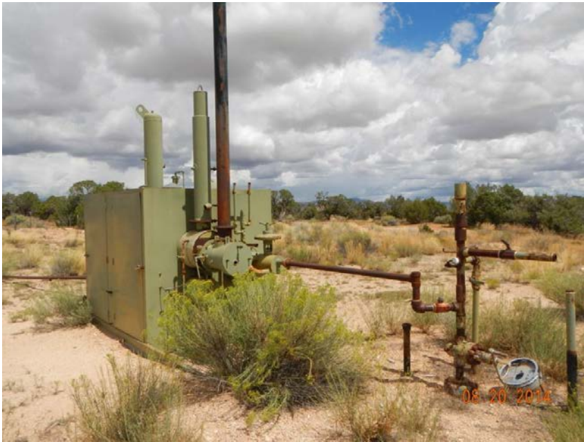
Photo 5. Horizontal heated separator. 39.323197/ -109.015442. Taken 8/20/14
