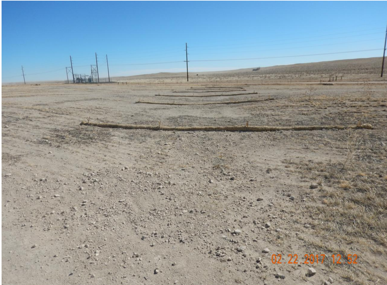
Photo 1: Photo taken from the south end of the location, facing south. Photo shows additional stormwater and sediment control BMPs have been installed in the interim area.
