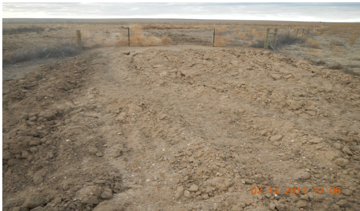
photo 4: Facing northwest toward the location. The location is fenced and soils have been ripped and partially contoured.
