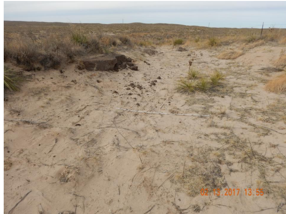
Photo 8: Photo taken from the east end of the location, facing north. Photo shows portions of the access road on location have not been reclaimed per reclamation rules. Erosion evident. Dark, stained soil exists and will need to be remediated. 6' measuring stick for reference.
