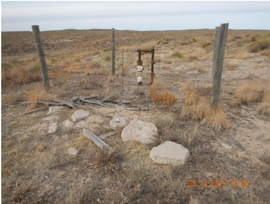
Photo 10: Photo taken from the southeast end of the location, facing north. Photo shows pipe riser, fence and debris remaining on location. Inspection Doc. # 673709790 identified this as a “Gasline tie/well”. Equipment and debris need to be removed.
