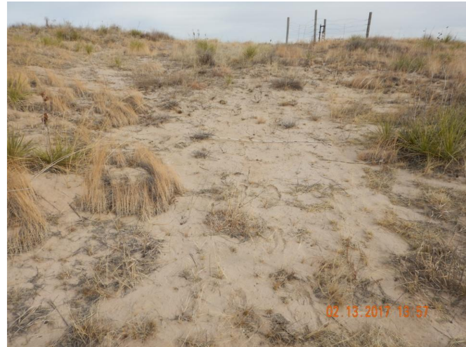
Photo 6: Photo taken from the west facing slope on the east end of the location, facing east. Photo shows areas of location that has not been stabilized, erosion evident. Photo also shows areas of location remain predominantly bare and exposed soil
