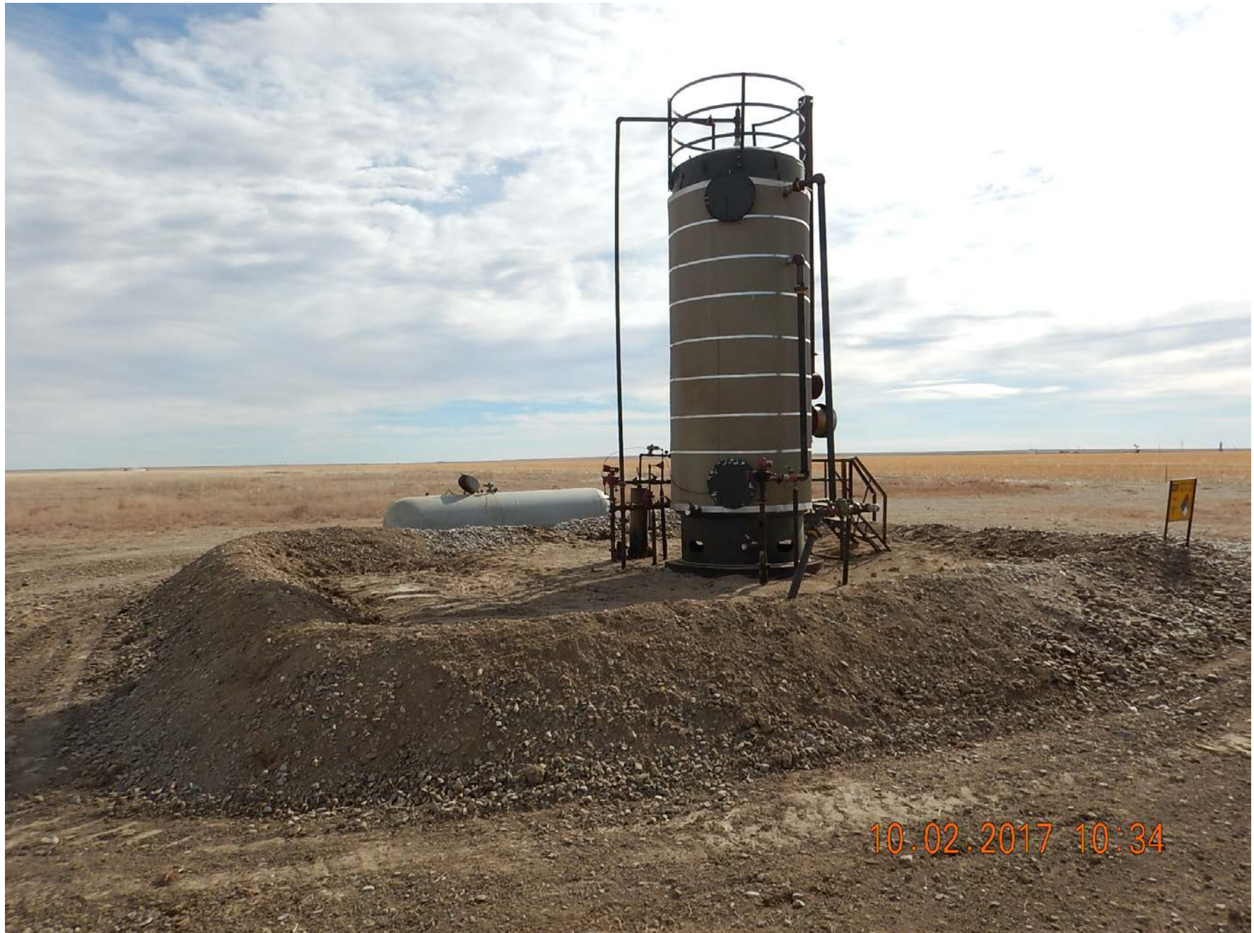
Heater treater where spill occurred. Spill was contained entirely within secondary containment according to Form 19.
