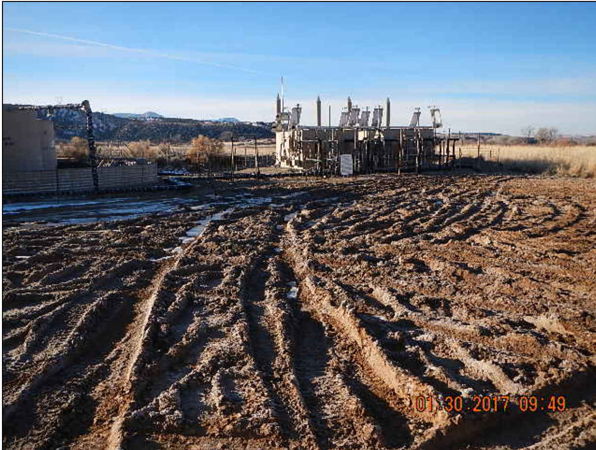
Photo 1. Rutting on location. No CA at time of inspection
