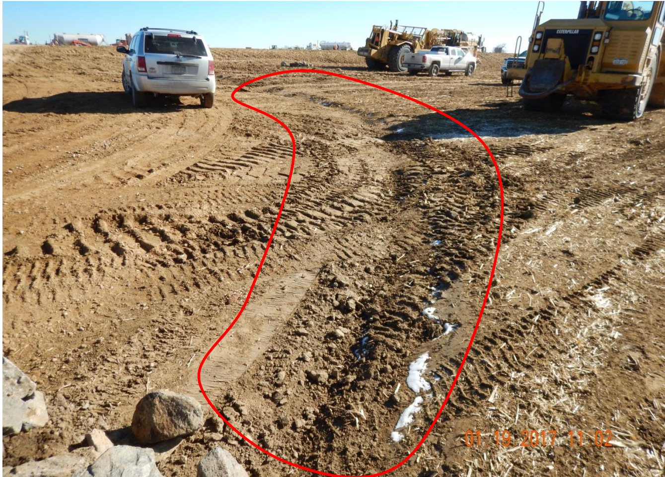
Photo 3. Photo taken from the western location, facing East. Equipment traffic should be kept off BMPs to ensure BMP properly functions. Need to maintain BMPs at all times.
