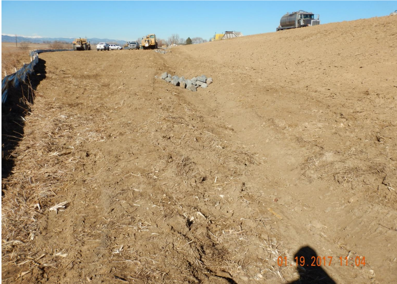
Photo 4. Photo taken from the western location, facing North. Silt fence, ditch and check dam BMPs installed. Fill slope appears to compacted and stabilized.
