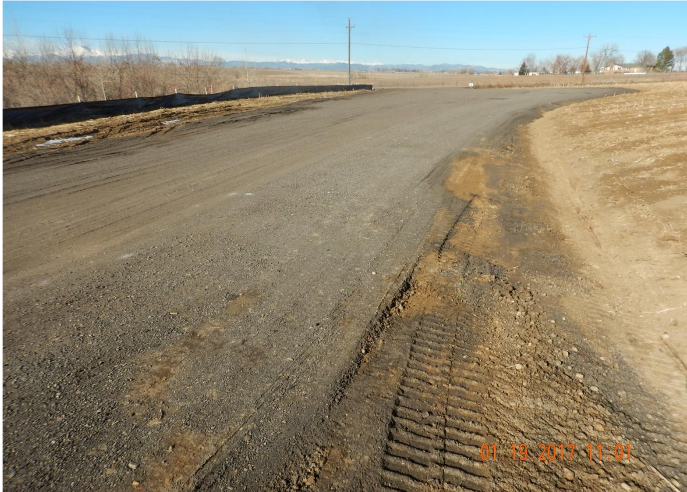
Photo 1. Photo taken from the entrance of location, facing Northwest. Vehicle tracking pad BMP installed. Did not observe any vehicle tracking onto the public road. Silt fence BMP installed at the entrance of location which extends to the southwest corner of location. A ditch- shallow along portions of the western location- and berm, and check dams installed around the perimeter of the location.
