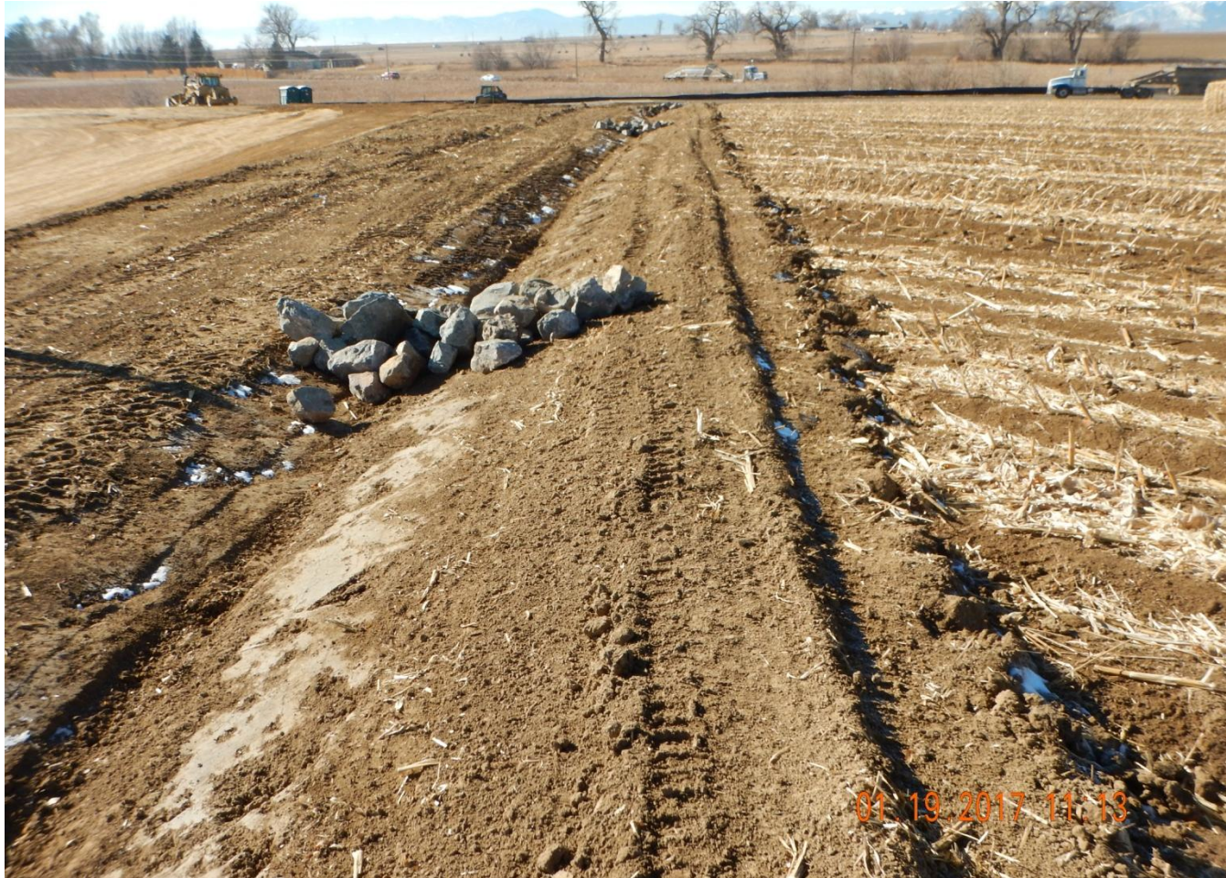
Photo 11. Photo taken from the northern location, facing Southwest. Ditch and berm BMP installed in conjunction with check dams.
