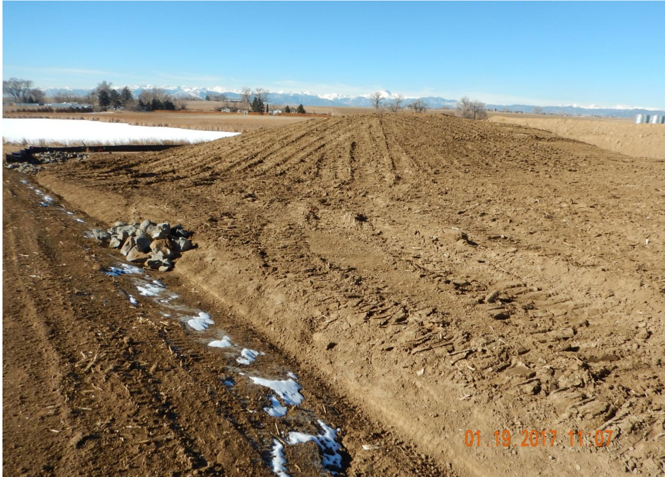
Photo 7. Photo taken from the southwest location, facing West. Topsoil stockpile stored along southwest location and temporarily stabilized (i.e., tracked).
