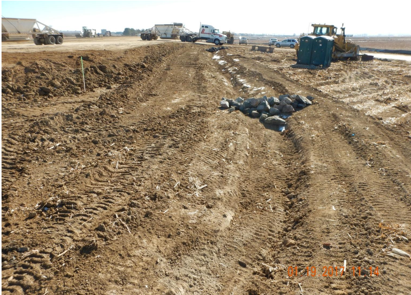
Photo 12. Photo taken from the northwest location, facing South. Ditch and berm BMP installed in conjunction with check dams.
