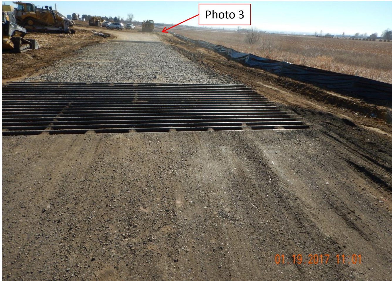
Photo 2. Photo taken from the entrance of location, facing Southwest. Vehicle tracking pad and device BMPs installed.
