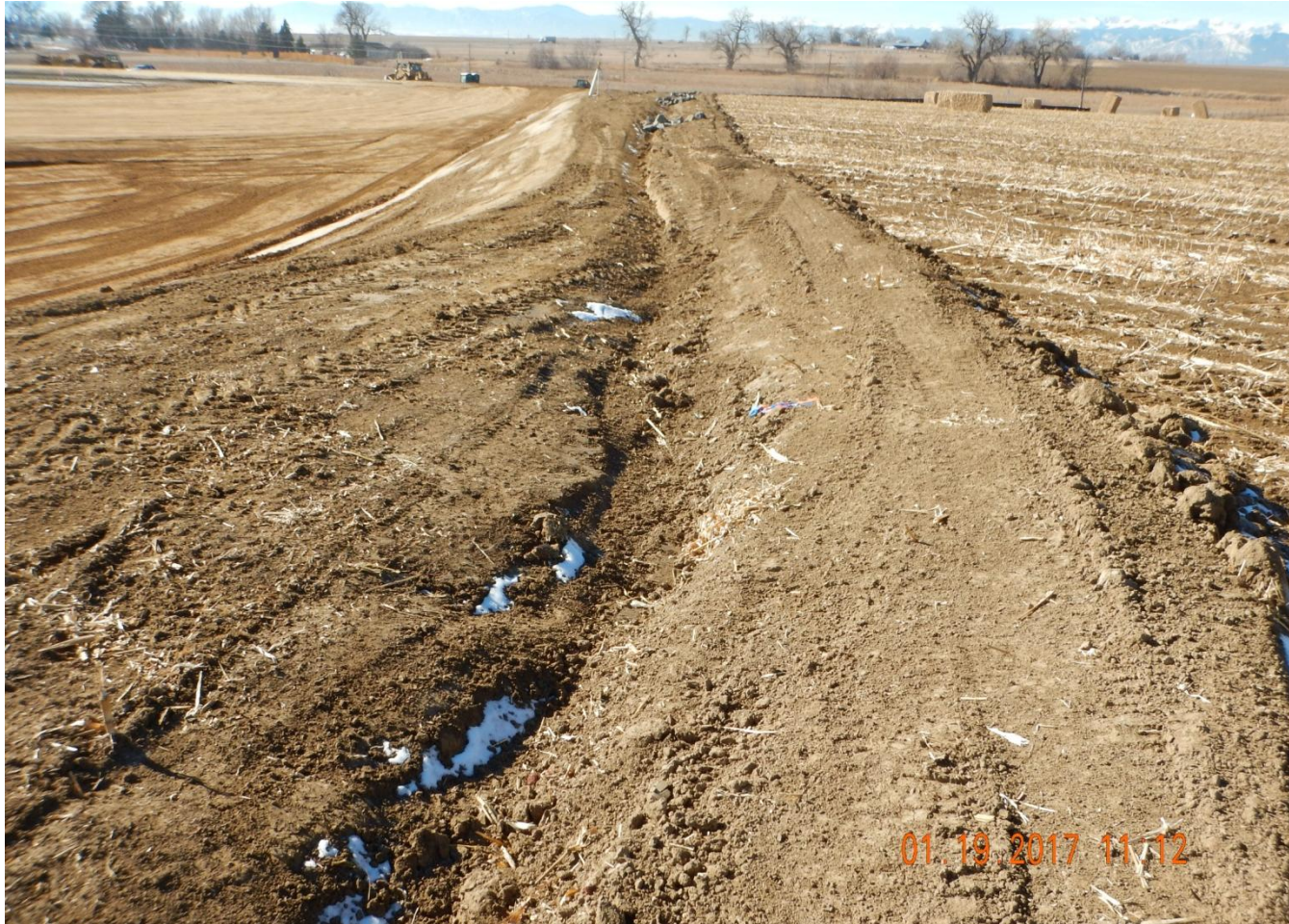
Photo 10. Photo taken from the northeast location, facing Southwest. Ditch and berm BMP installed in conjunction with check dams.
