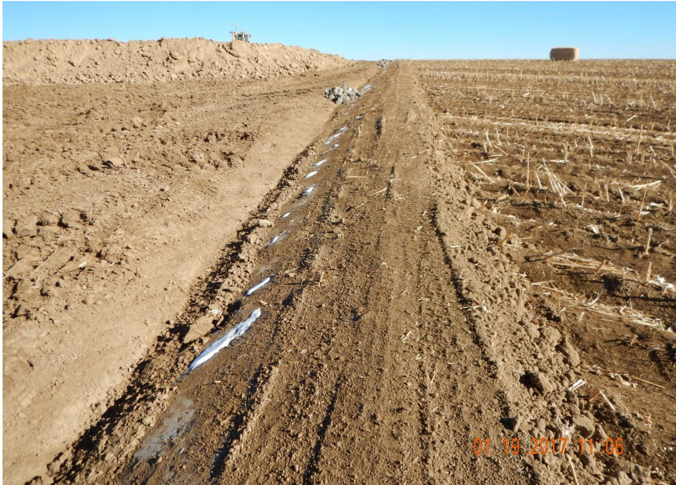
Photo 6. Photo taken from the southwest location, facing Northeast. Ditch and berm BMP installed in conjunction with check dams. Location IN-PROCESS of being stabilized. Fill slope still needs to be stabilized.
