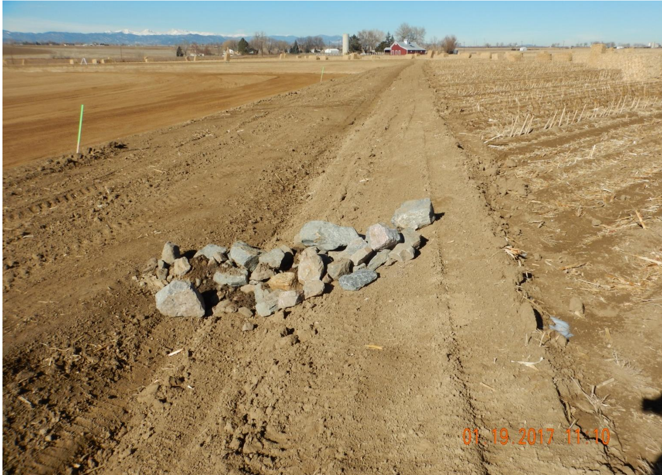
Photo 9. Photo taken from the eastern location, facing Northwest. Ditch and berm BMP installed in conjunction with check dams.
