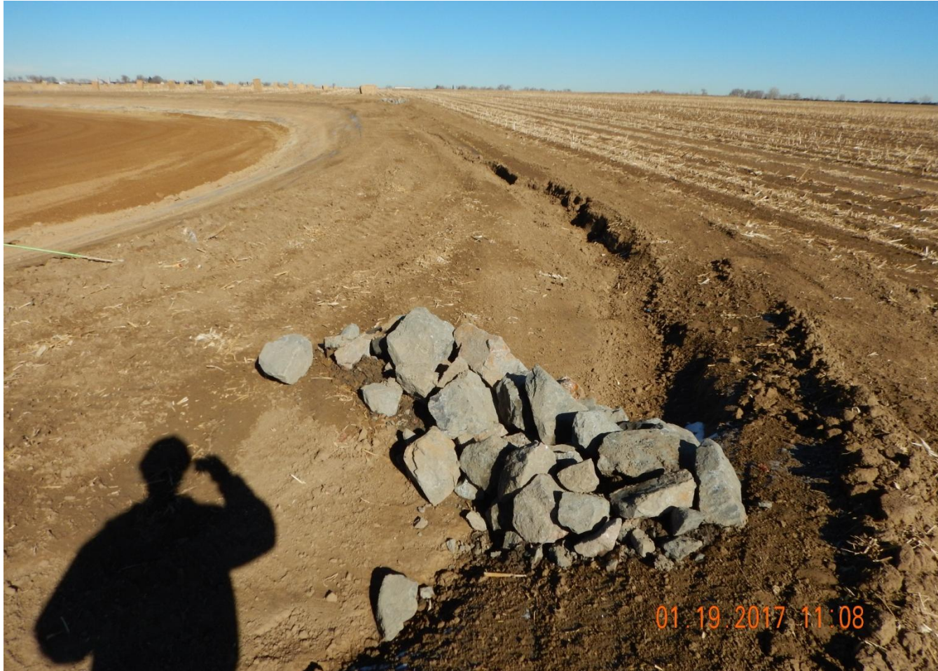
Photo 8. Photo taken from the southeast location, facing North. Ditch and berm BMP installed in conjunction with check dams. Cut slope along the southeast, east and northeast location appear to be stabilized.
