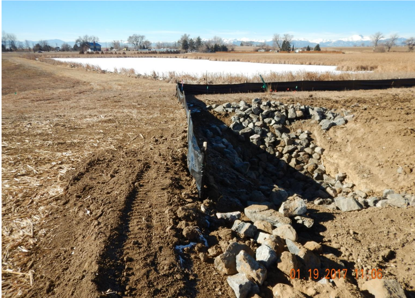
Photo 5. Photo taken from the southwest location, facing West. Sediment trap lined and stabilized in conjunction with silt fence.
