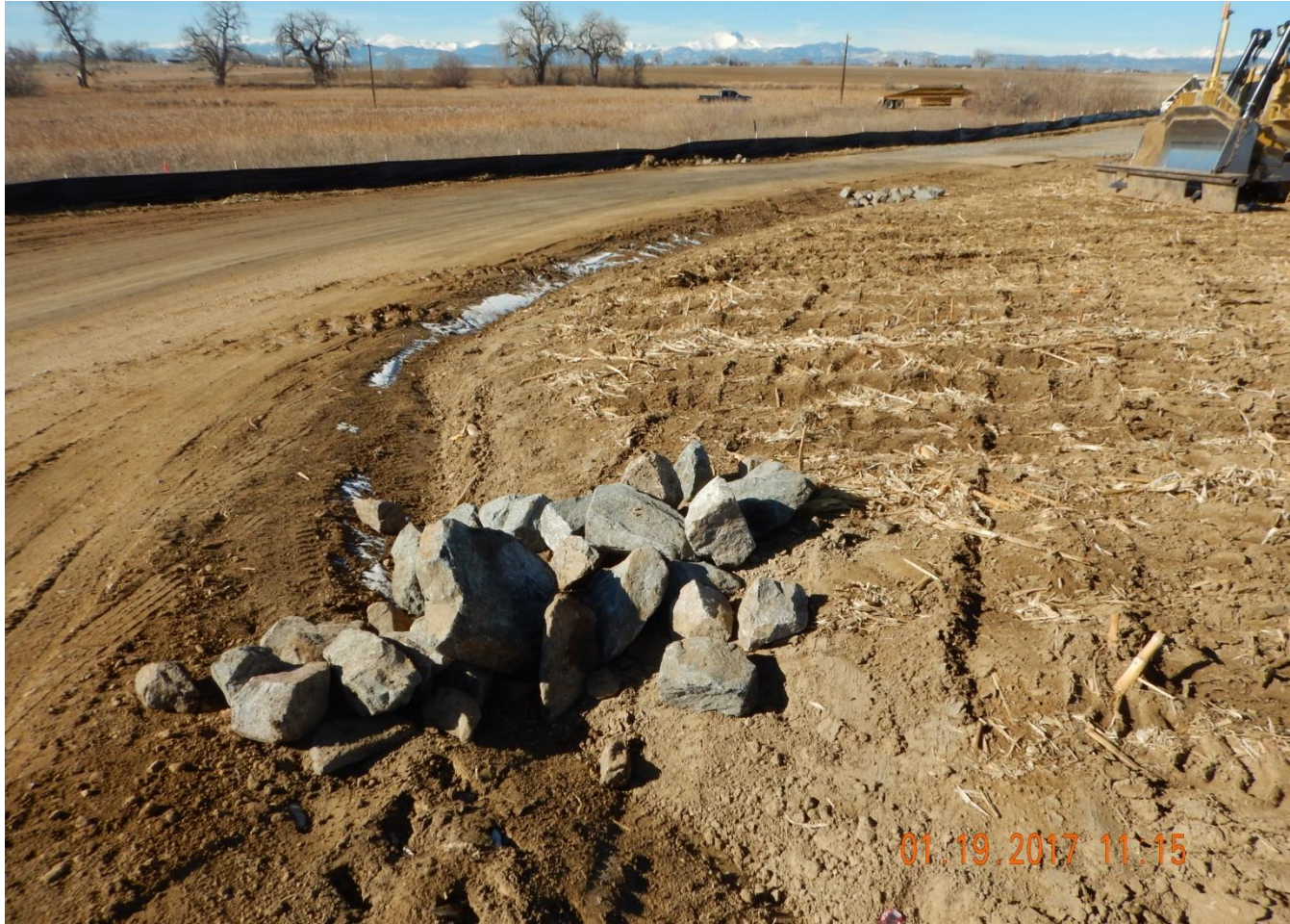
Photo 13. Photo taken from the western location, facing West. Ditch and berm BMP installed in conjunction with check dams.
