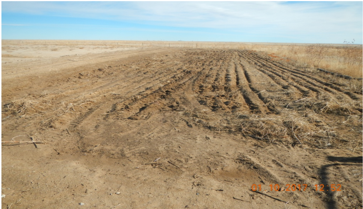
photo 3: The soils have been ripped around the location for surface roughening BMP.
