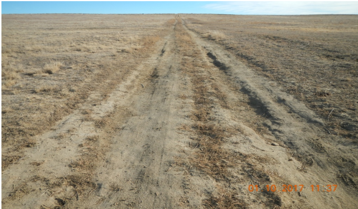
photo 5: Facing east along the access road. This are signs of vehicle rutting in this area.
