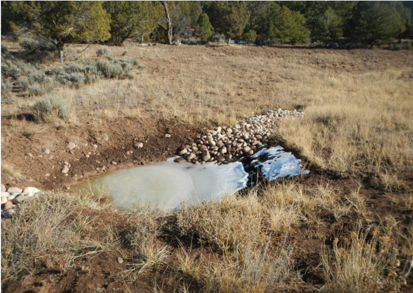
Photo 8. View of newly installed silt trap in the northern portion of the project area. Overflow and a portion of diversion channel are lined with cobble.
