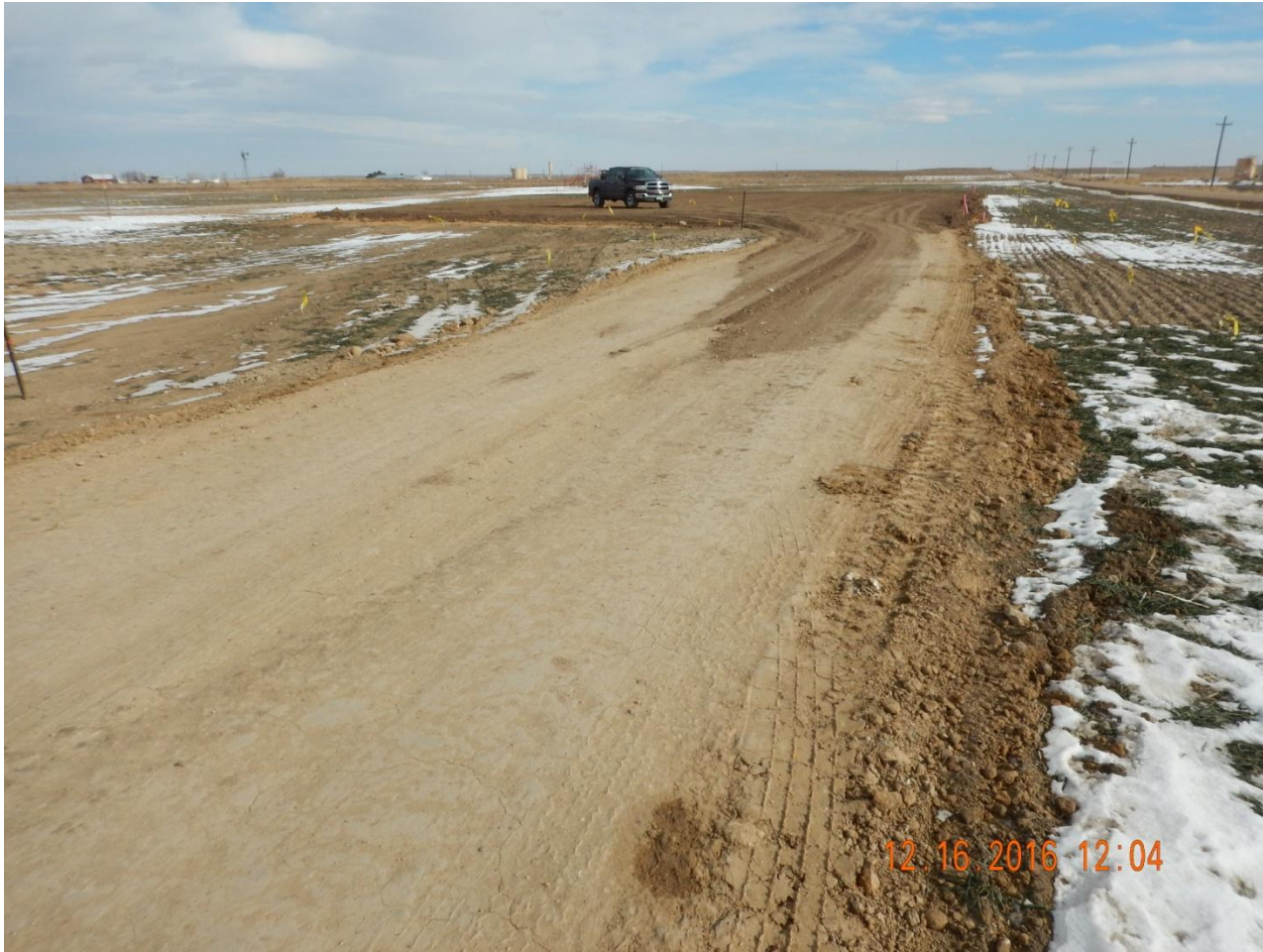
Photo 1. Photo taken from the entrance of location, facing East. Location IN-PROCESS of being built. Topsoil was not salvaged before construction of location. Also, no stormwater or erosion control BMPs in place prior to or during construction.
