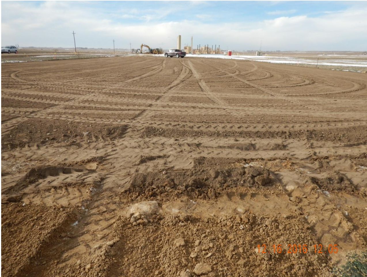
Photo 2. Photo taken from the eastern location, facing West. Location IN-PROCESS of being built. Topsoil was not salvaged before construction of location. Also, no stormwater or erosion control BMPs in place prior to or during construction.
