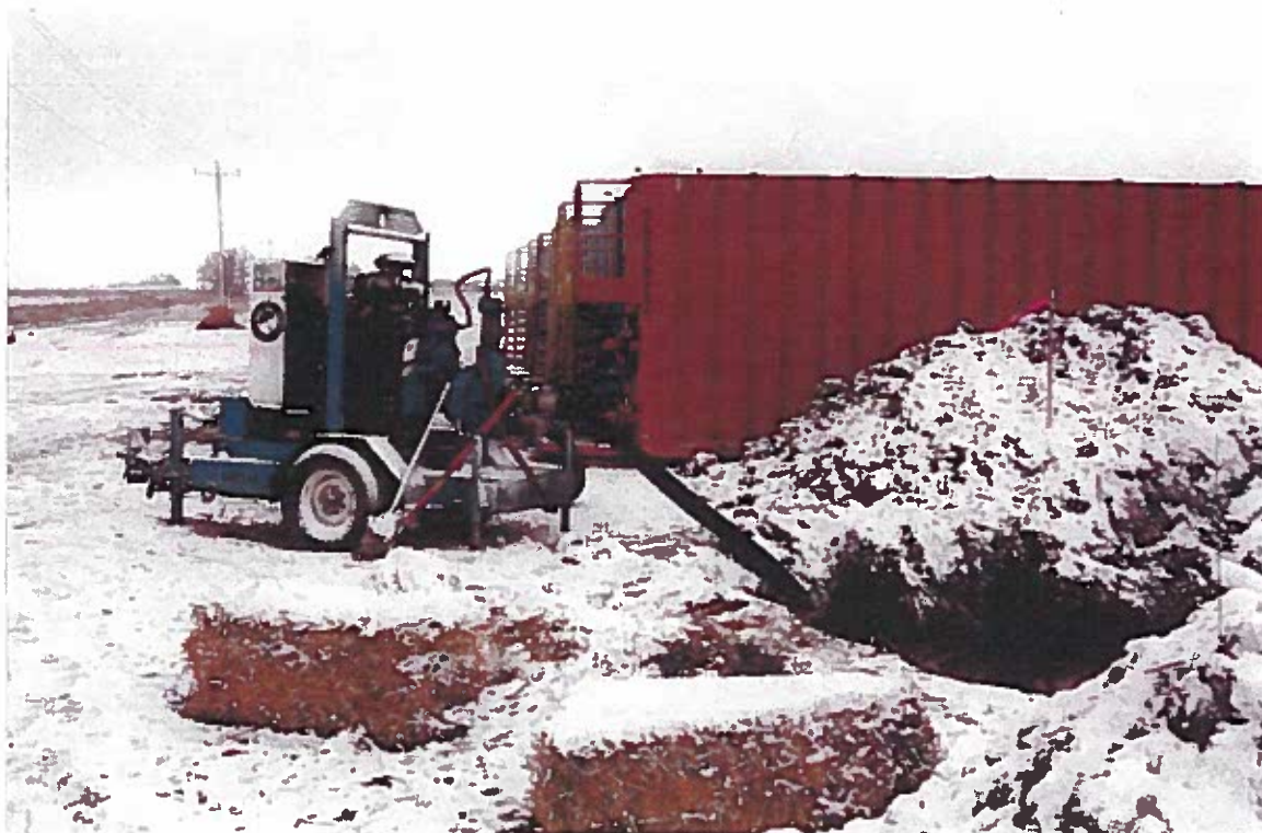
Photo 7 - Petro-Canada dug and excavation to recover water draining from the farm field drainage system. A large capacity pump moved recovered waste liquids into frac tanks.
