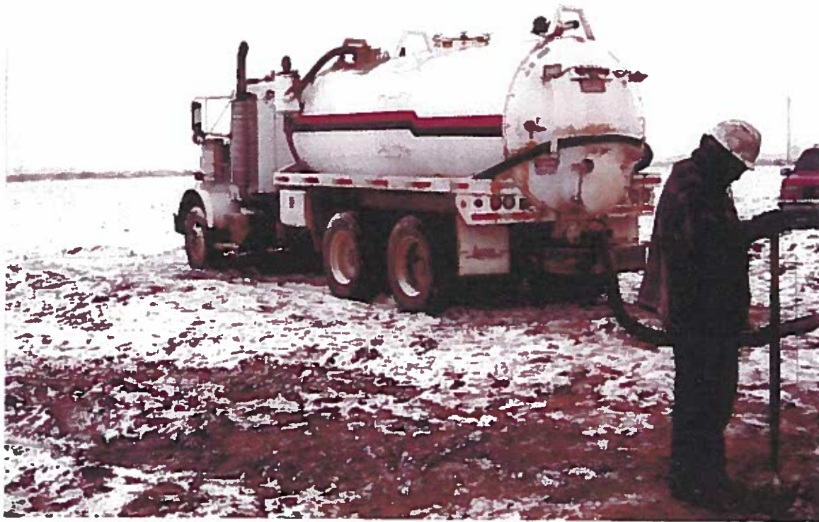
Photo 5 - A vacuum truck recovers ground water from a test excavation.
