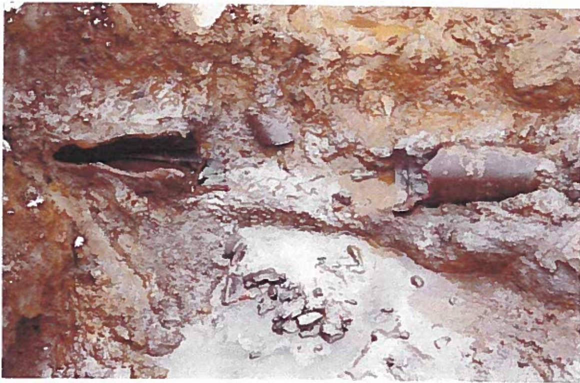
Photo 2 - Photograph of broken field drainage tile. The drainage system is buried 6 feet below grade.
