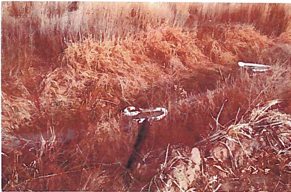
Photo 6 - Oil sorbent booms were placed into a nearby irrigation ditch.
