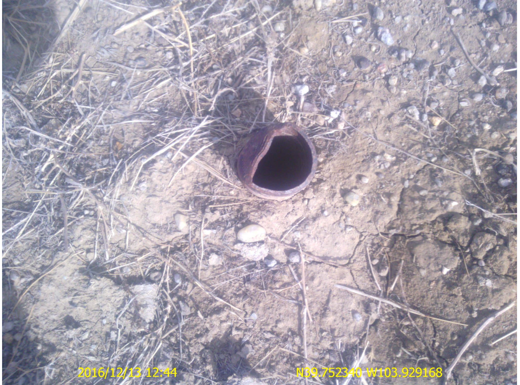
Figure 8: Photo taken from the west end of the location. Photo shows exposed pipe remaining in the ground
