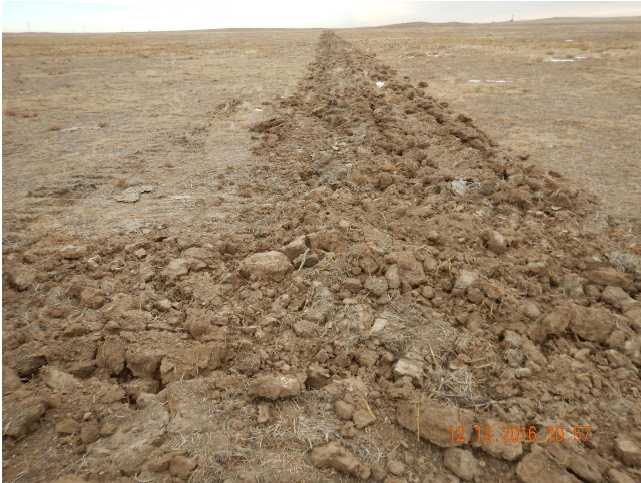
Photo 3. Photo taken from the southwest location, facing East. Temporary BMP, surface roughening, installed around perimeter of location before construction of the location.
