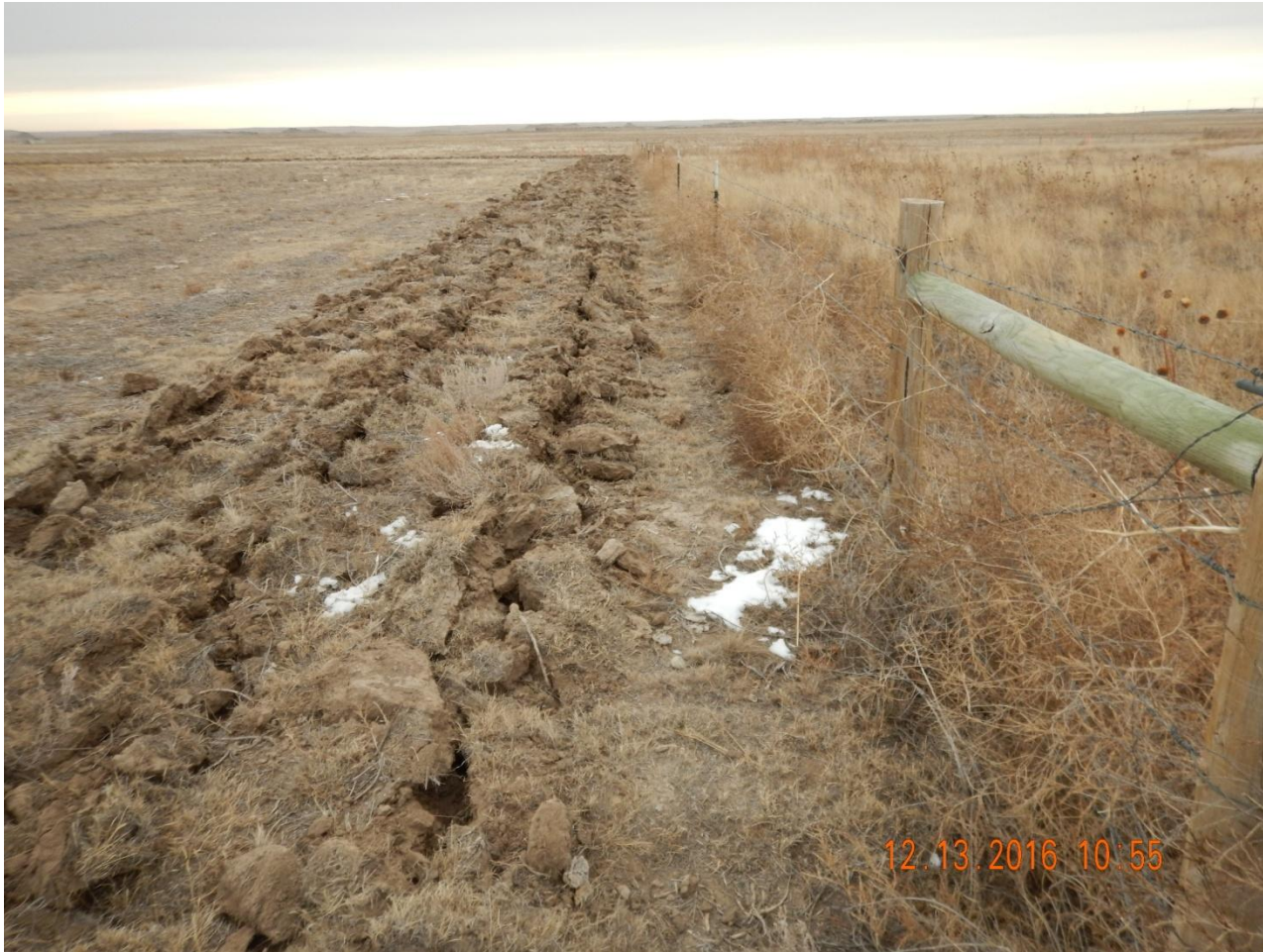
Photo 2. Photo taken from the western location, facing South. Temporary BMP, surface roughening, installed around perimeter of location before construction of the location.
