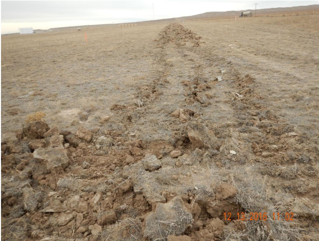
Photo 5. Photo taken from the northeast location, facing West. Temporary BMP, surface roughening, installed around perimeter of location before construction of the location.
