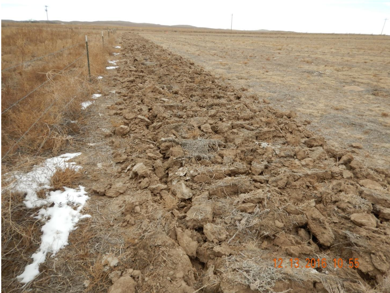
Photo 1. Photo taken from the western location, facing North. Temporary BMP, surface roughening, installed around perimeter of location before construction of the location.
