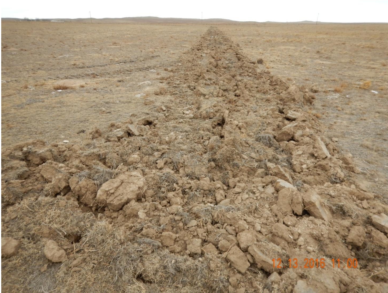
Photo 4. Photo taken from the southeast location, facing North. Temporary BMP, surface roughening, installed around perimeter of location before construction of the location.
