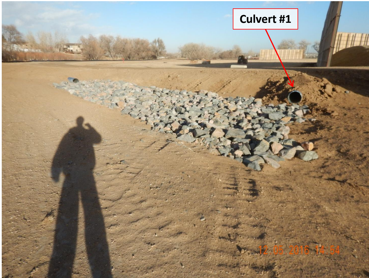
Photo 3. Photo taken from the entrance of the well location, facing East. Area has been stabilized to control sediment laden storm runoff from leaving location.
