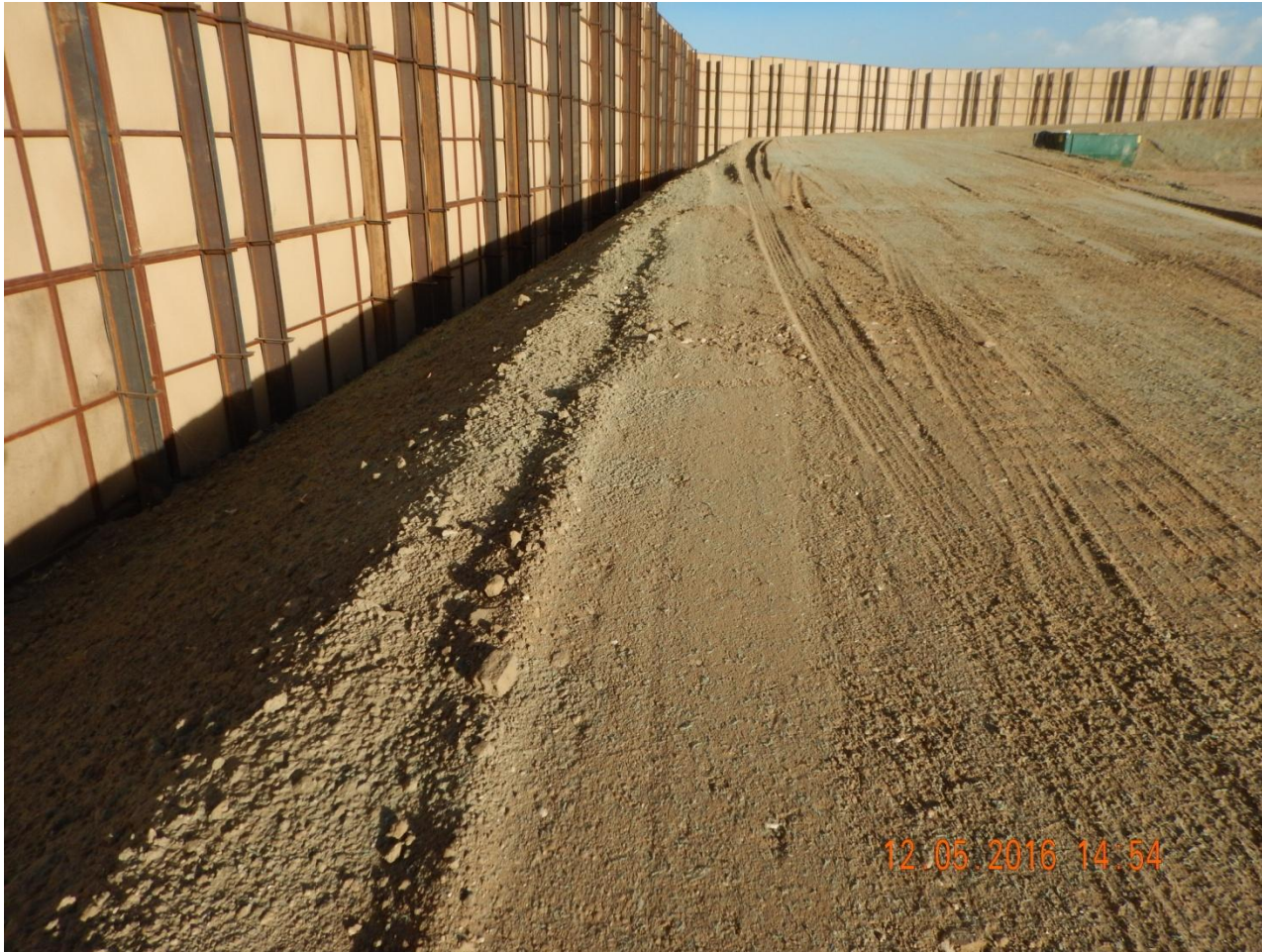
Photo 6. Photo taken from the entrance of the location, facing East, along the inside perimeter soil barrier. Soil barrier and MLVT area has been sprayed with a tacifier to stabilize from erosion.
