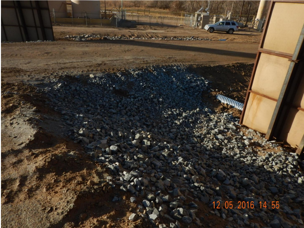
Photo 5. Photo taken from the east-side of the entrance of the well location, facing West. Fill slope has been stabilized to prevent erosion.
