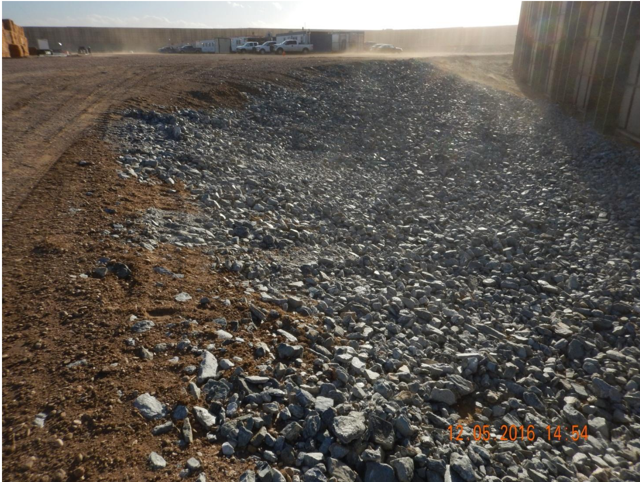
Photo 4. Photo taken from the west-side of the entrance of the well location, facing South. Fill slope has been stabilized to prevent erosion.
