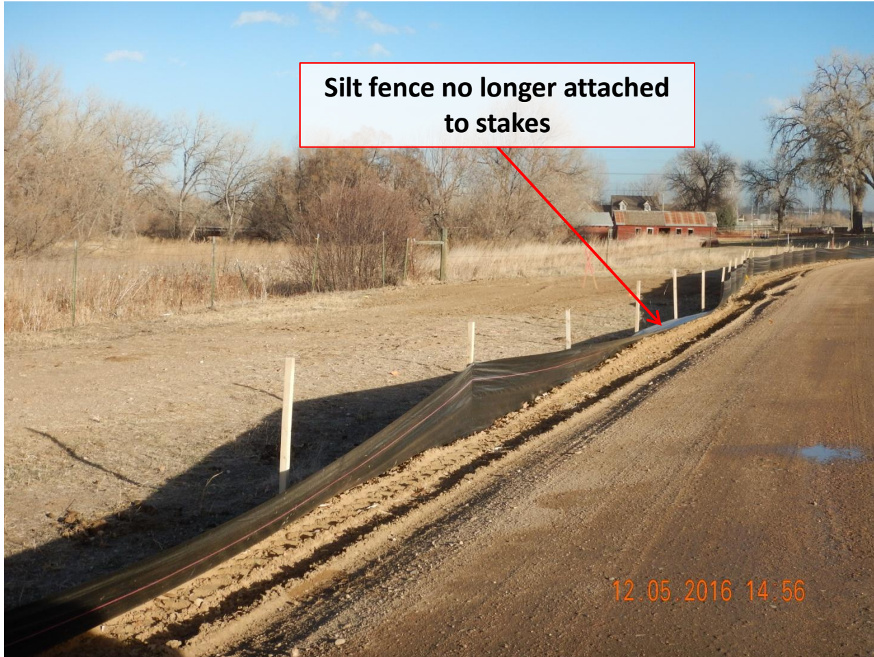
Photo 7. Photo taken from the access road near the entrance of the location, facing East. Silt fence has been installed along the northern portion of the access road and needs to be maintained.
