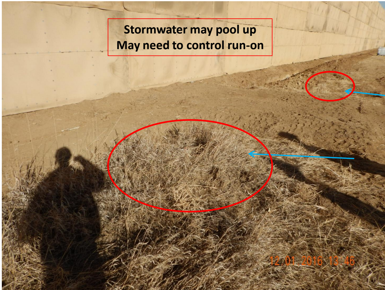
Photo 1. Photo taken from the southern location, along the existing access road, facing East. Stormwater from the existing access road will likely travel north towards location and pool up in red-circled areas. May need to control stormwater run-on.
