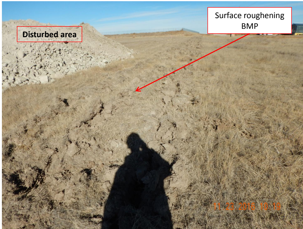
Photo 6. Photo taken from the southeast Tombstone pad, facing North. Surface roughening BMP, which is a temporary BMP, was installed during this inspection.
