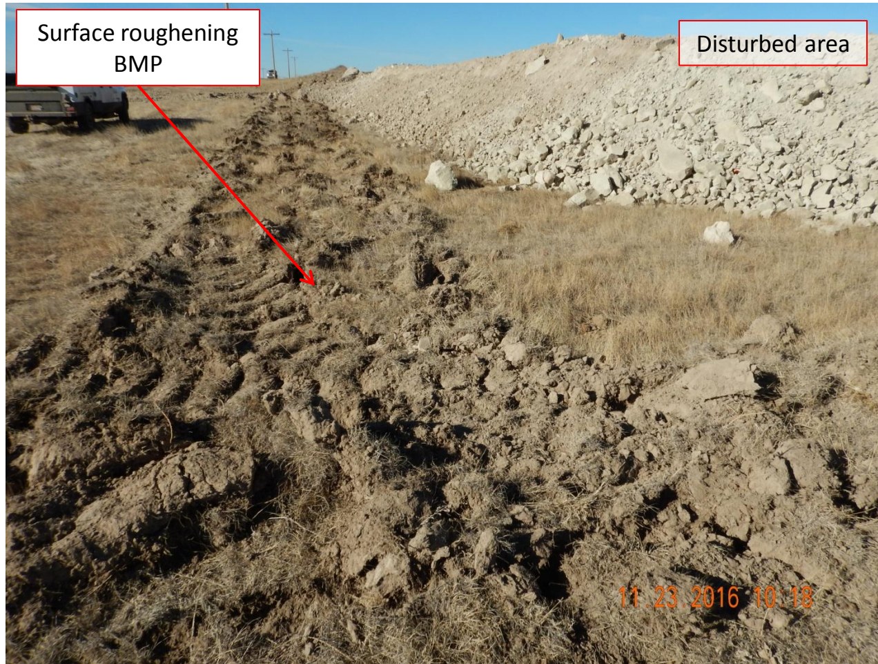
Photo 5. Photo taken from the southeast Tombstone pad, facing West. Surface roughening BMP, which is a temporary BMP, was installed during this inspection.
