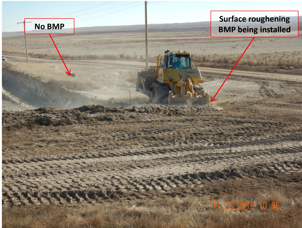
Photo 2. Photo taken from the previous location, facing East, towards the southern Tombstone pad. After making a previous call to the operator regarding a location ~ ¼ mile to the west that did not have stormwater and erosion control BMPs, a BMP was installed during this inspection.
