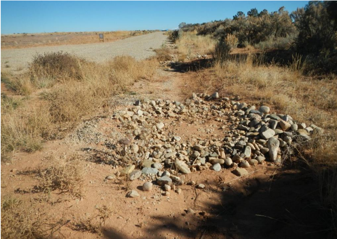
Photo 5. View of stormwater controls along the southern edge of the well pad and access road that appear to be functioning.
