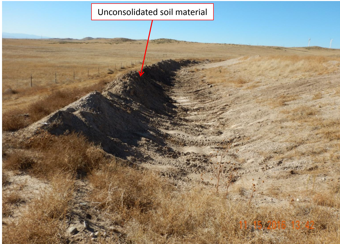
Photo 3. Photo taken from entrance of location, facing West. Need to stabilize unconsolidated soil material and implement BMPs in accordance with good engineering practices along the southern location in a manner that minimizes erosion, transport of sediment offsite, and site degradation per Rule 1002.f.
