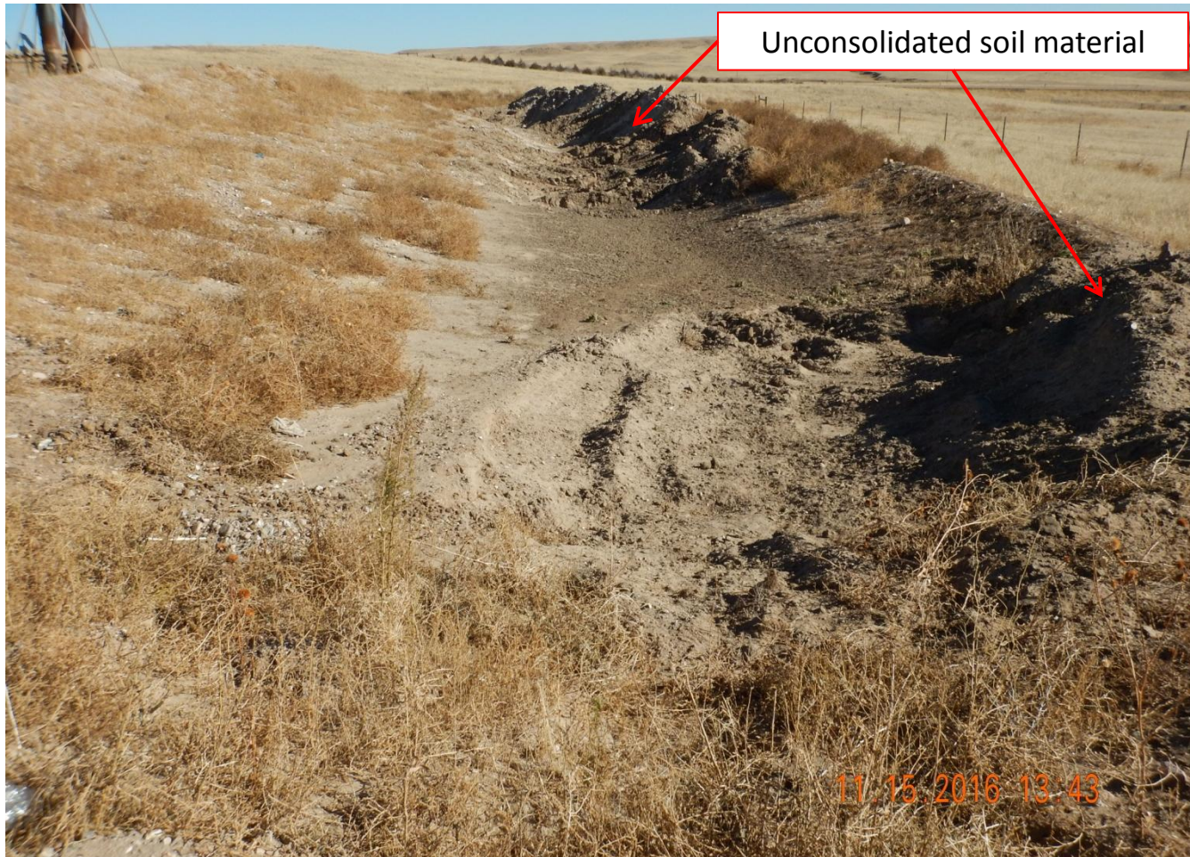
Photo 4. Photo taken from entrance of location, facing East. Need to stabilize unconsolidated soil material and implement BMPs in accordance with good engineering practices along the southern location in a manner that minimizes erosion, transport of sediment offsite, and site degradation per Rule 1002.f.
