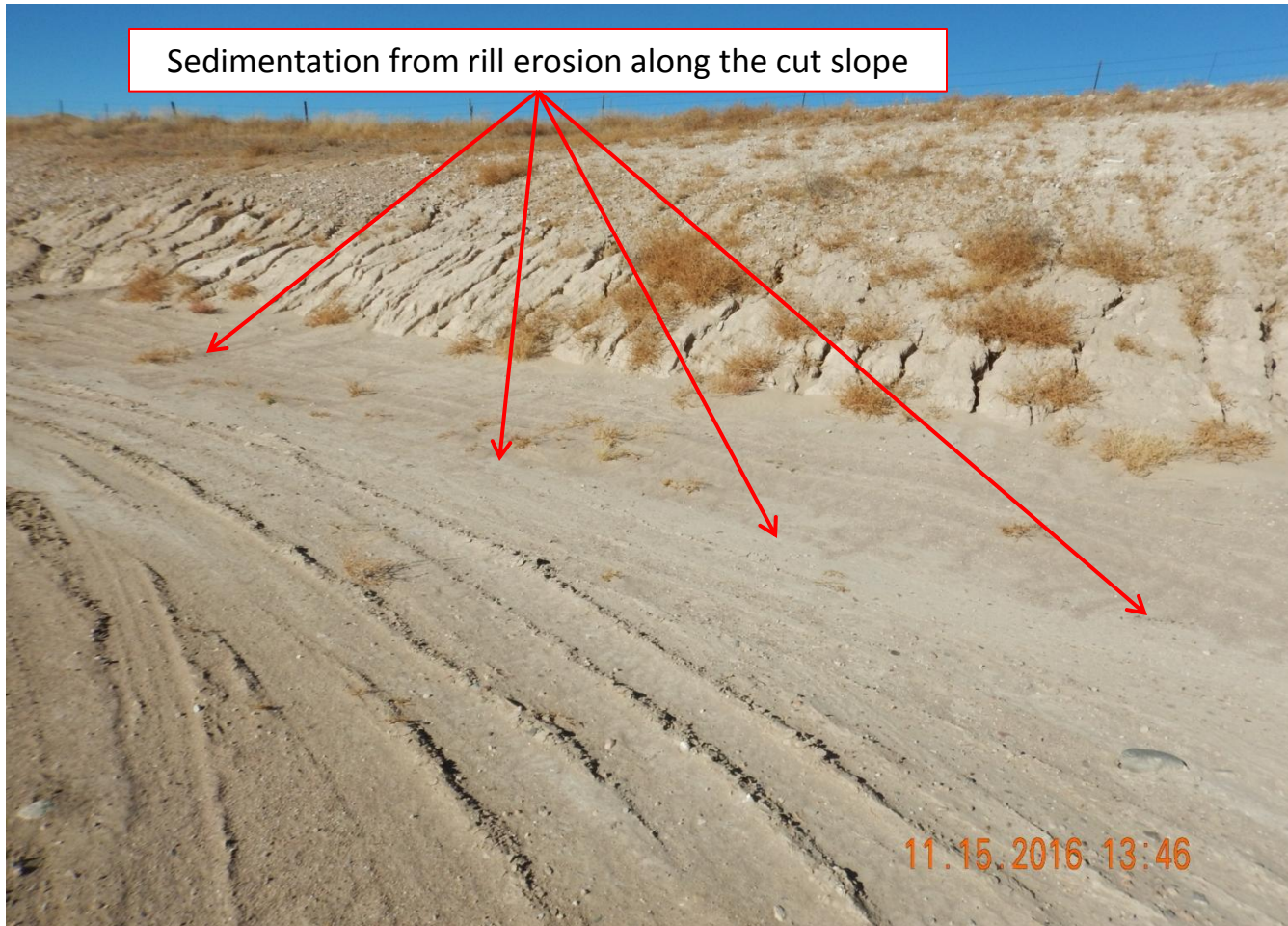
Photo 5. Photo taken from the northeast location, facing North. Rill erosion occurring throughout entire north cut slope. Need to stabilize and implement erosion controls designed to minimize erosion along the entire north cut slope per Rule 1002.f.
