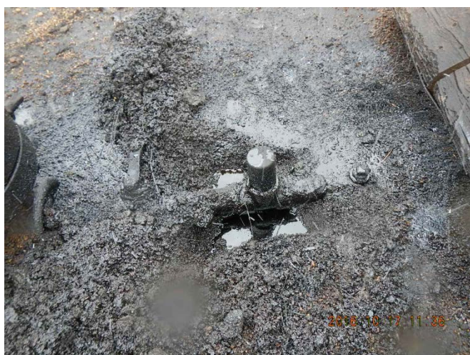
057-06062 possible bull plug leak.
