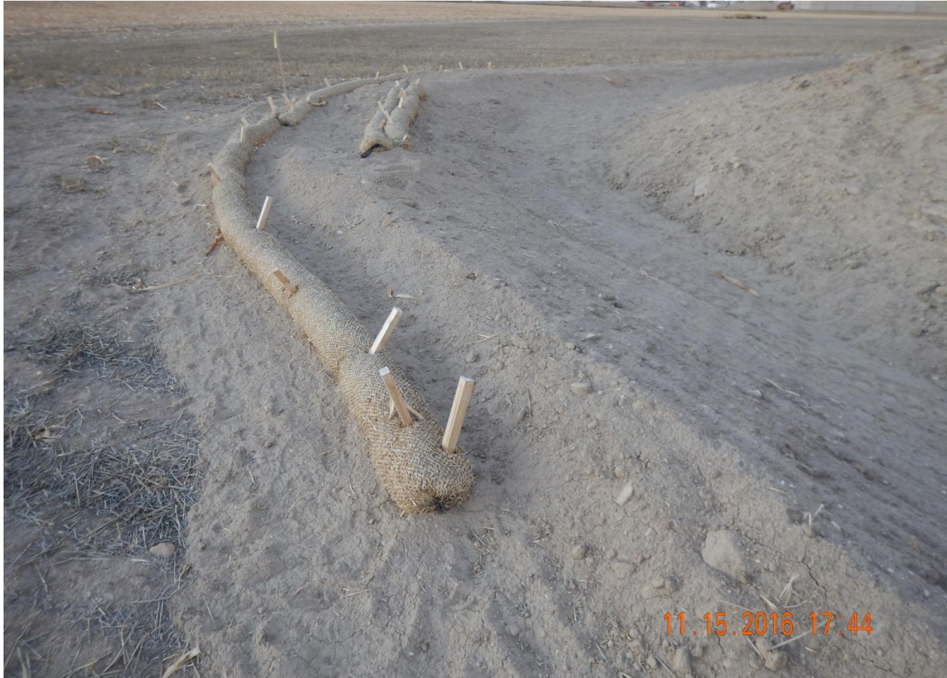
Photo 1. Photo taken from the western location, facing North. Installed wattles along the potential discharge point.
