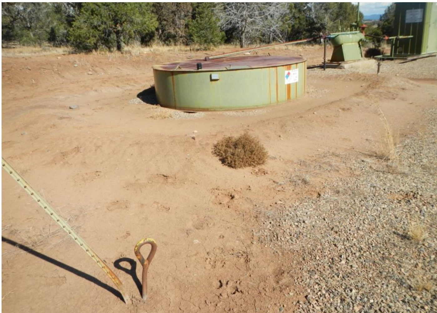
Photo 6. View of tank berm that is no longer functioning.
