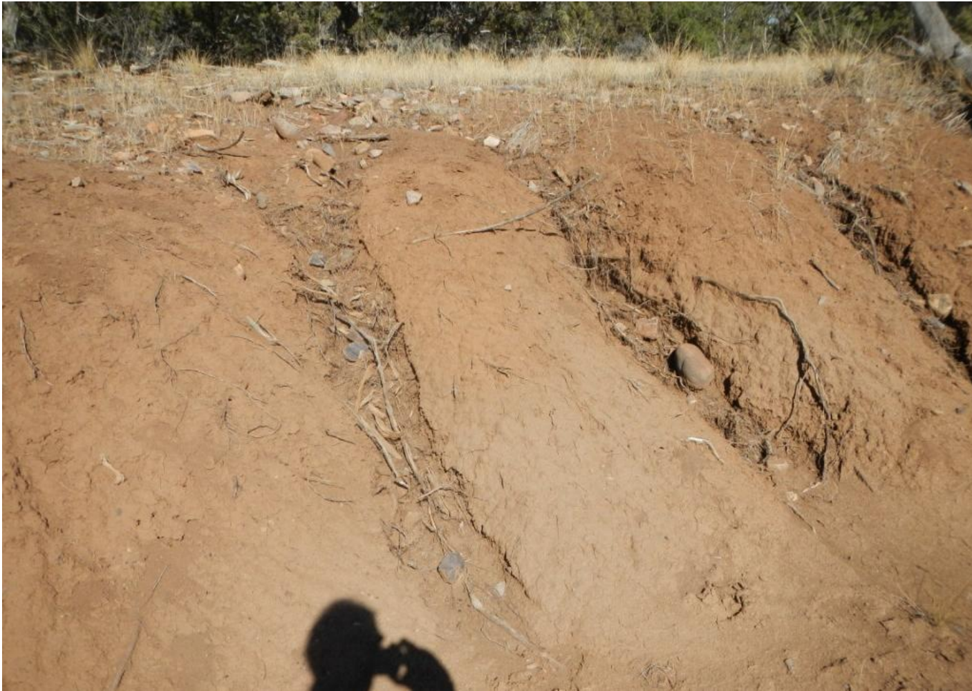
Photo 7. View of erosion exposing roots from adjacent vegetation within the eastern edge of the well pad cut-slope. Stormwater flows are eroding cut-slopes from stormwater run-on and slopes need to be stabilized.
