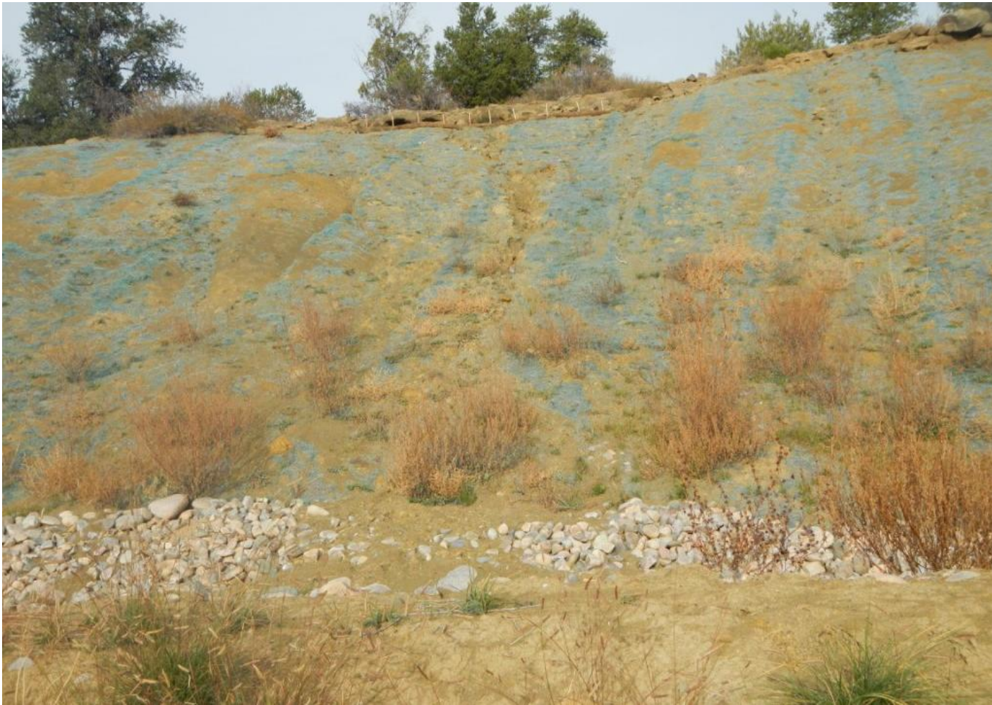
Photo 6. View of the northwestern portion of the project area. Revegetation is sparse on the slope. Stormwater erosion is occurring beneath the wattle at the top of the slope. This area needs maintenance and likely further stabilization to prevent further erosional channeling.
