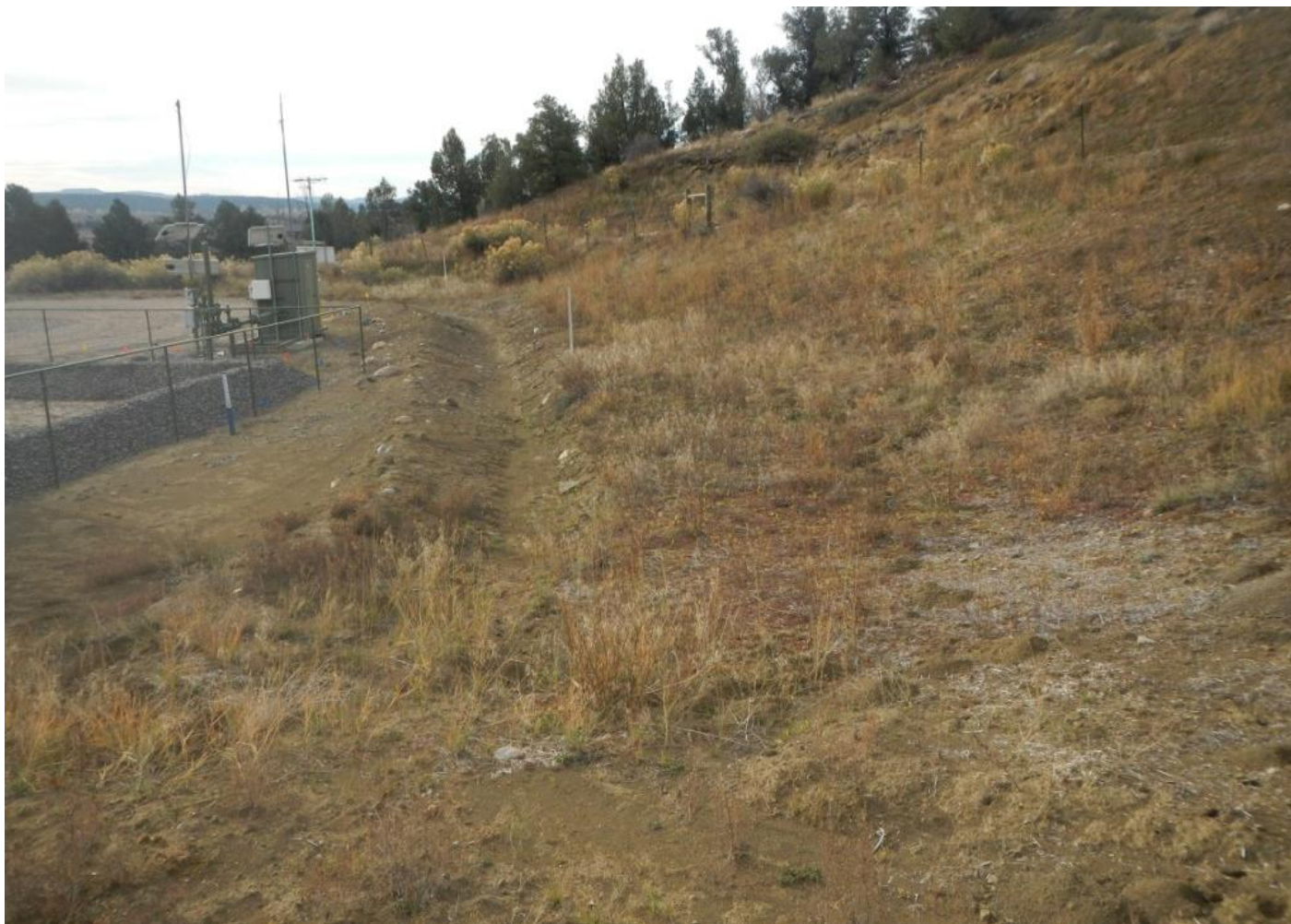
Photo 4. View of the southeastern portion of the project area. Revegetation is progressing on this slope and diversion is in good condition.
