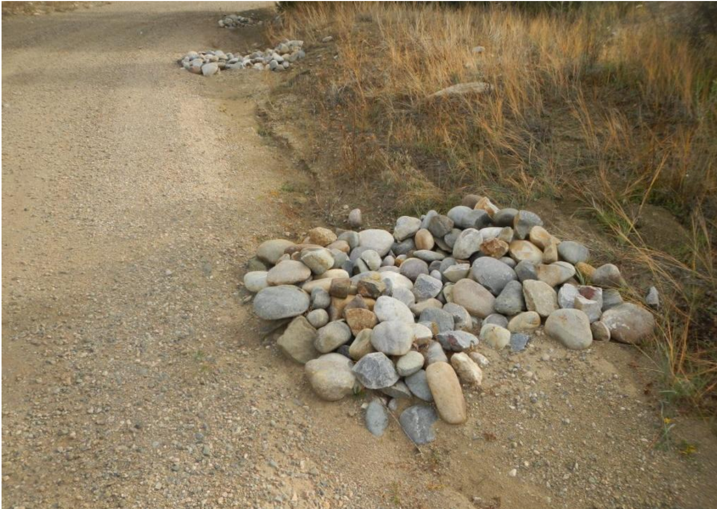
Photo 1. View of rock check dams on eastern edge of access that need maintenance.
