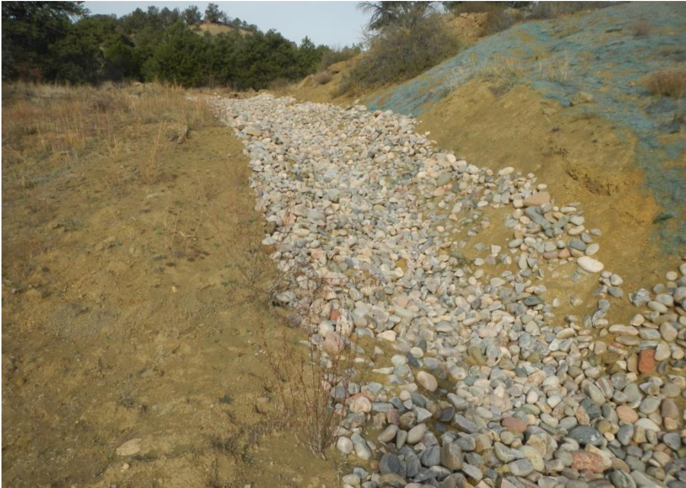
Photo 3. View of stormwater controls in the eastern portion of the project area. Appears to be functioning at this time.
