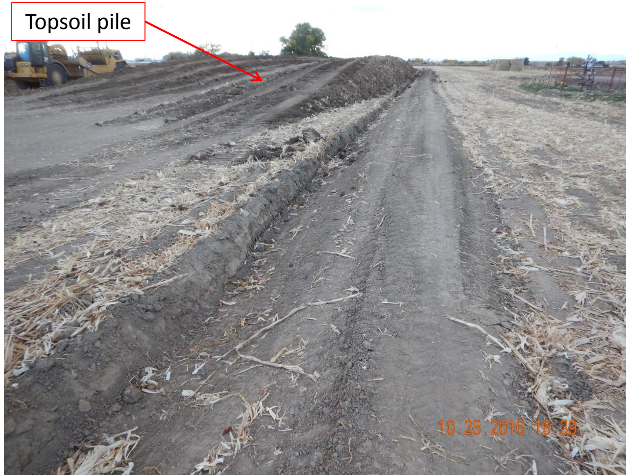
Photo 1. Photo taken from northern perimeter of location, facing West. Topsoil salvage IN-PROCESS and being stored along northern location. Ditch and berm constructed around outer perimeter of the location.
