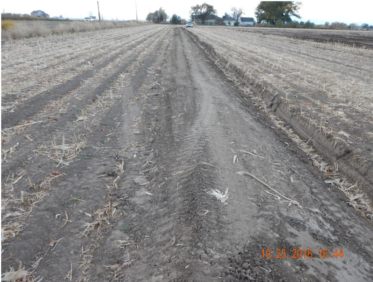
Photo 4. Photo taken from southern perimeter of location, facing West. Ditch and berm constructed around outer perimeter of the location.
