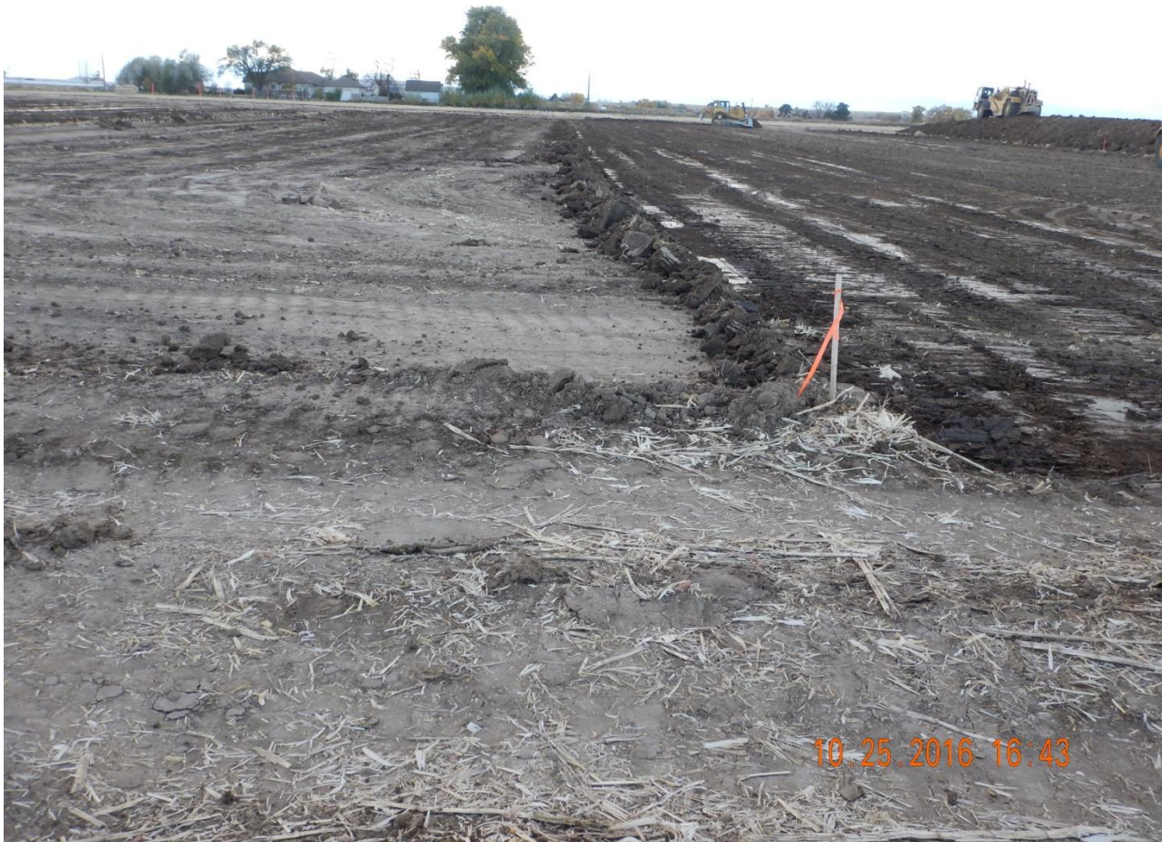
Photo 3. Photo taken from eastern perimeter of location, facing West. Topsoil salvage IN-PROCESS.
