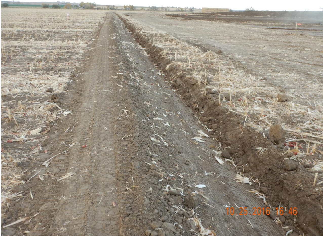
Photo 5. Photo taken from western perimeter of location, facing North. Ditch and berm constructed around outer perimeter of the location.
