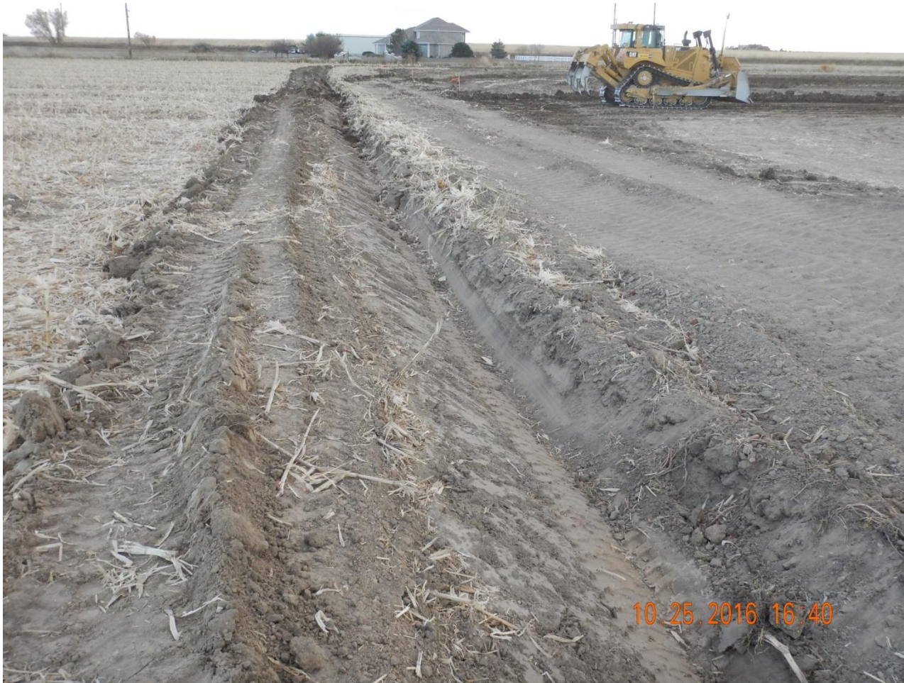
Photo 2. Photo taken from eastern perimeter of location, facing South. Ditch and berm constructed around outer perimeter of the location.
