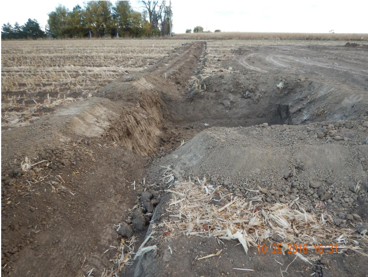
Photo 3. Photo taken from eastern perimeter of the location, facing South. Sediment trap installed which will be stabilized per the contractor. Ditch and berm constructed around outer perimeter of the location.
