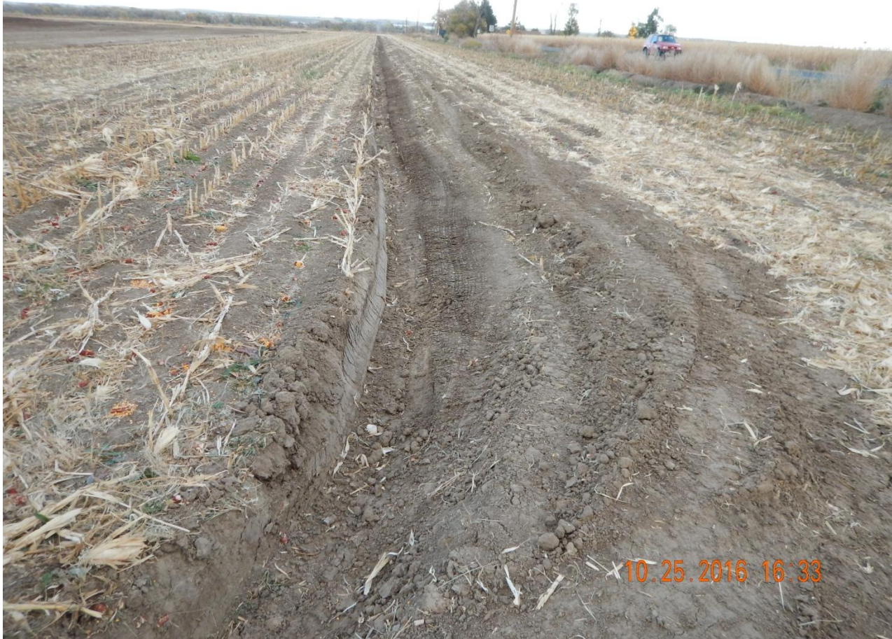
Photo 4. Photo taken from southwestern corner of perimeter, facing East. Ditch and berm constructed around outer perimeter of the location.
