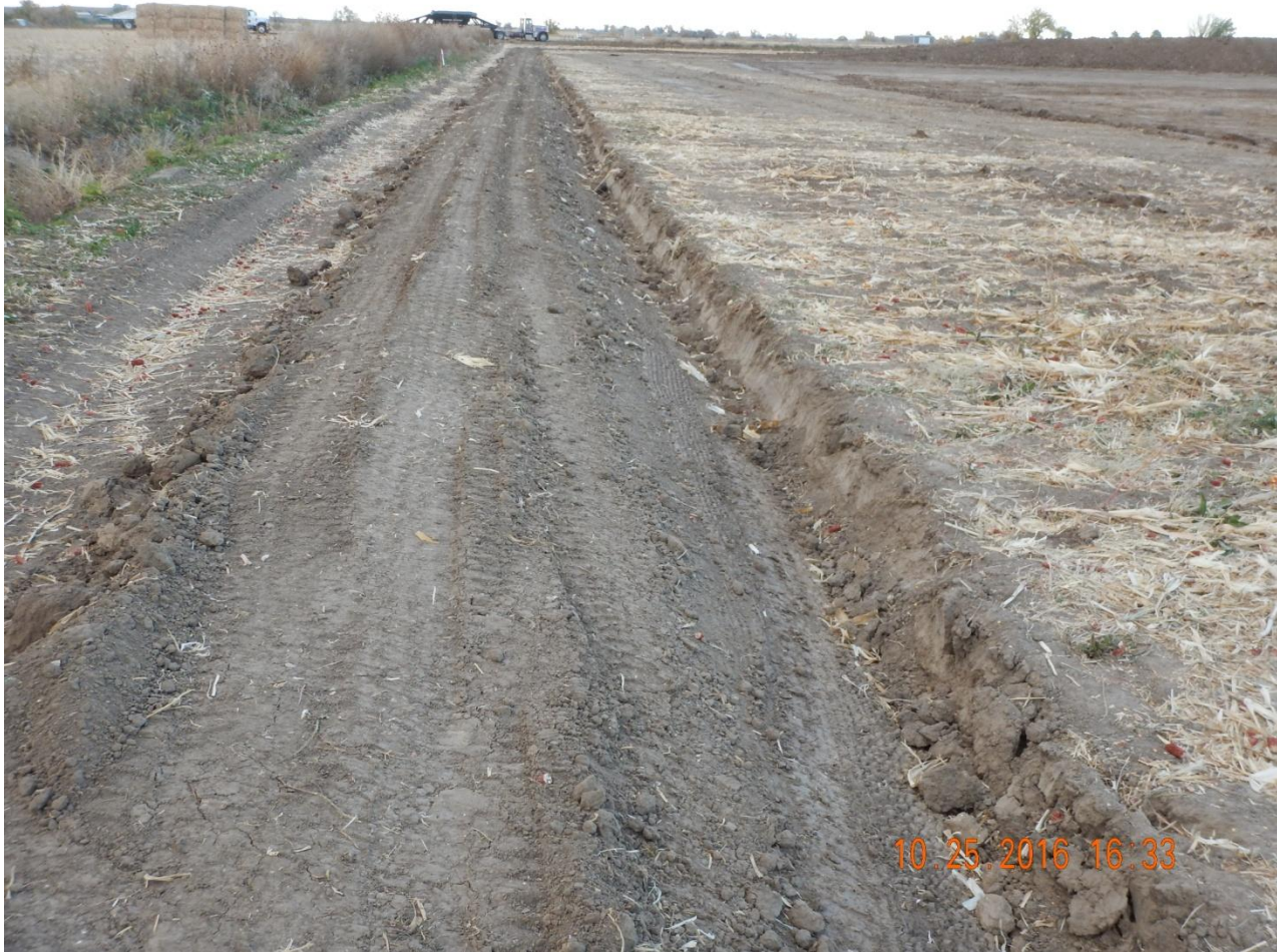
Photo 5. Photo taken from southwestern corner of perimeter, facing North. Ditch and berm constructed around outer perimeter of the location.
