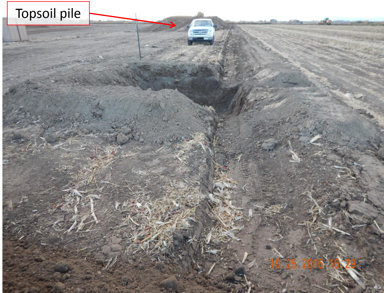
Photo 1. Photo taken from northeastern corner of perimeter, facing West. Sediment trap installed which will be stabilized per the contractor. Topsoil pile stored along northern location. Ditch and berm constructed around outer perimeter of the location.
