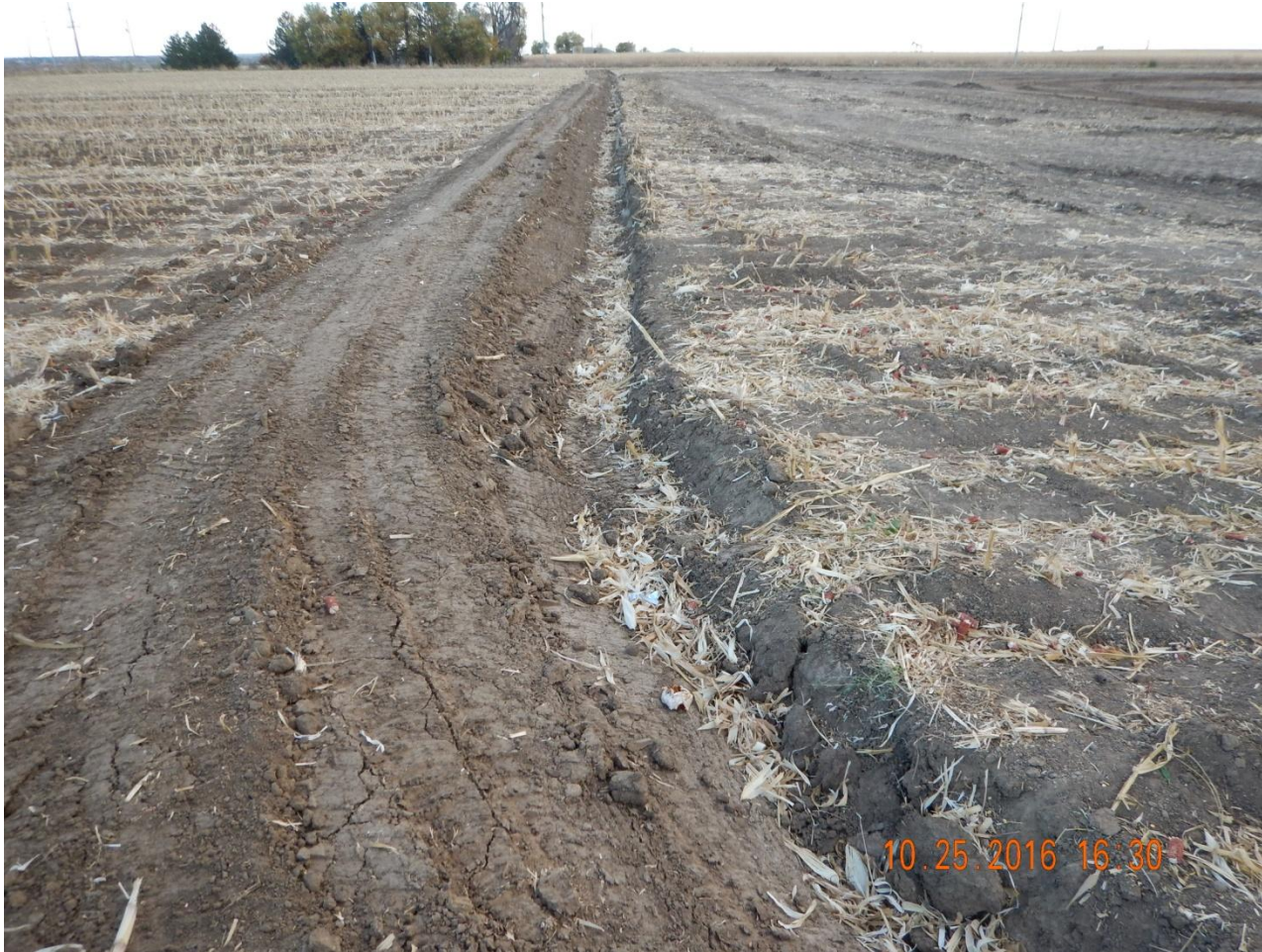
Photo 2. Photo taken from northeastern corner of perimeter, facing South. Ditch and berm constructed around outer perimeter of the location.
