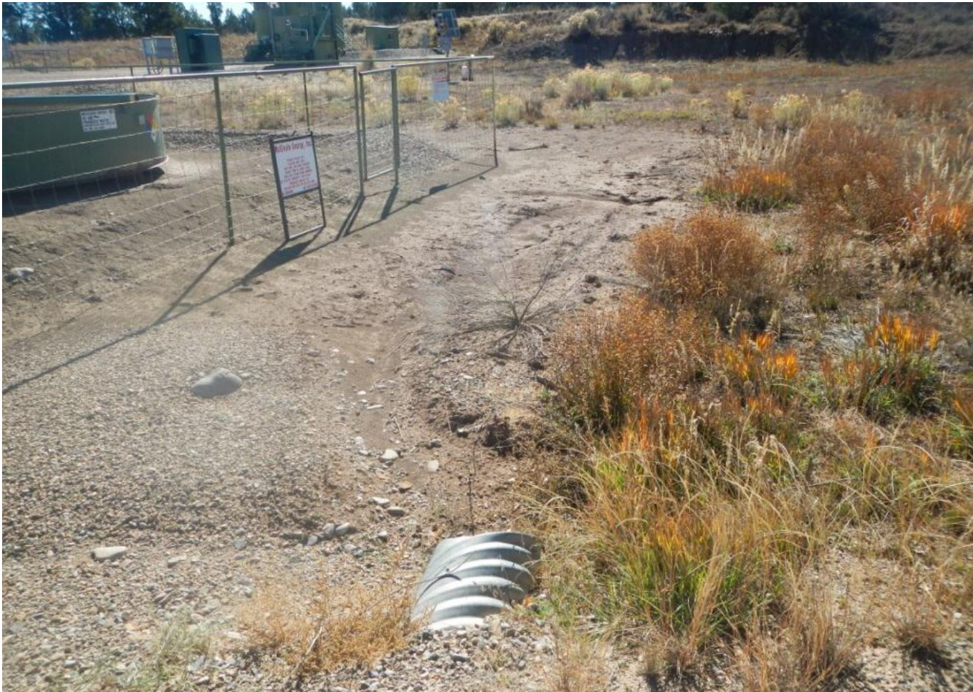
Photo 4. View of area where stormwater flows enter culvert and it appears sediment is carried with it.
