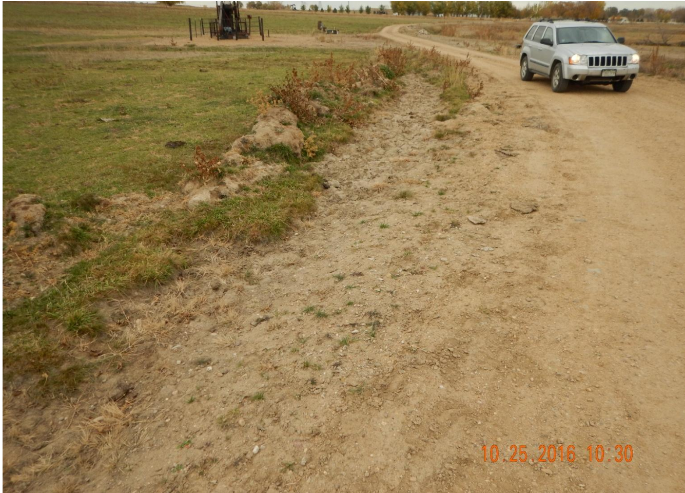
Photo 3. Photo taken north of the shared tank battery location, facing North along the access road. Need to repair access road that was widened by an operator and re-seed any portions that are disturbed during this process.
