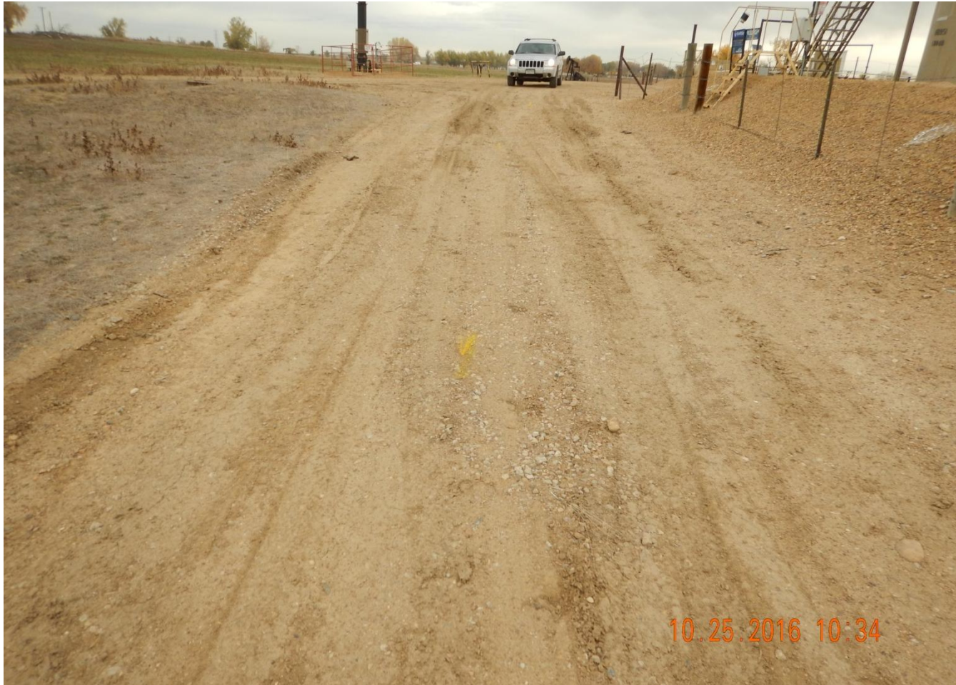
Photo 1. Photo taken west of the batteries, facing North. Corrective actions to repair ruts have been performed.
