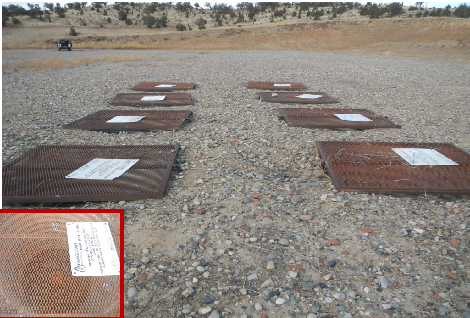
Photo#3: Eight Wells on Location have been P&A'd; Insert; view of Plated welded on Cut off Casing.
