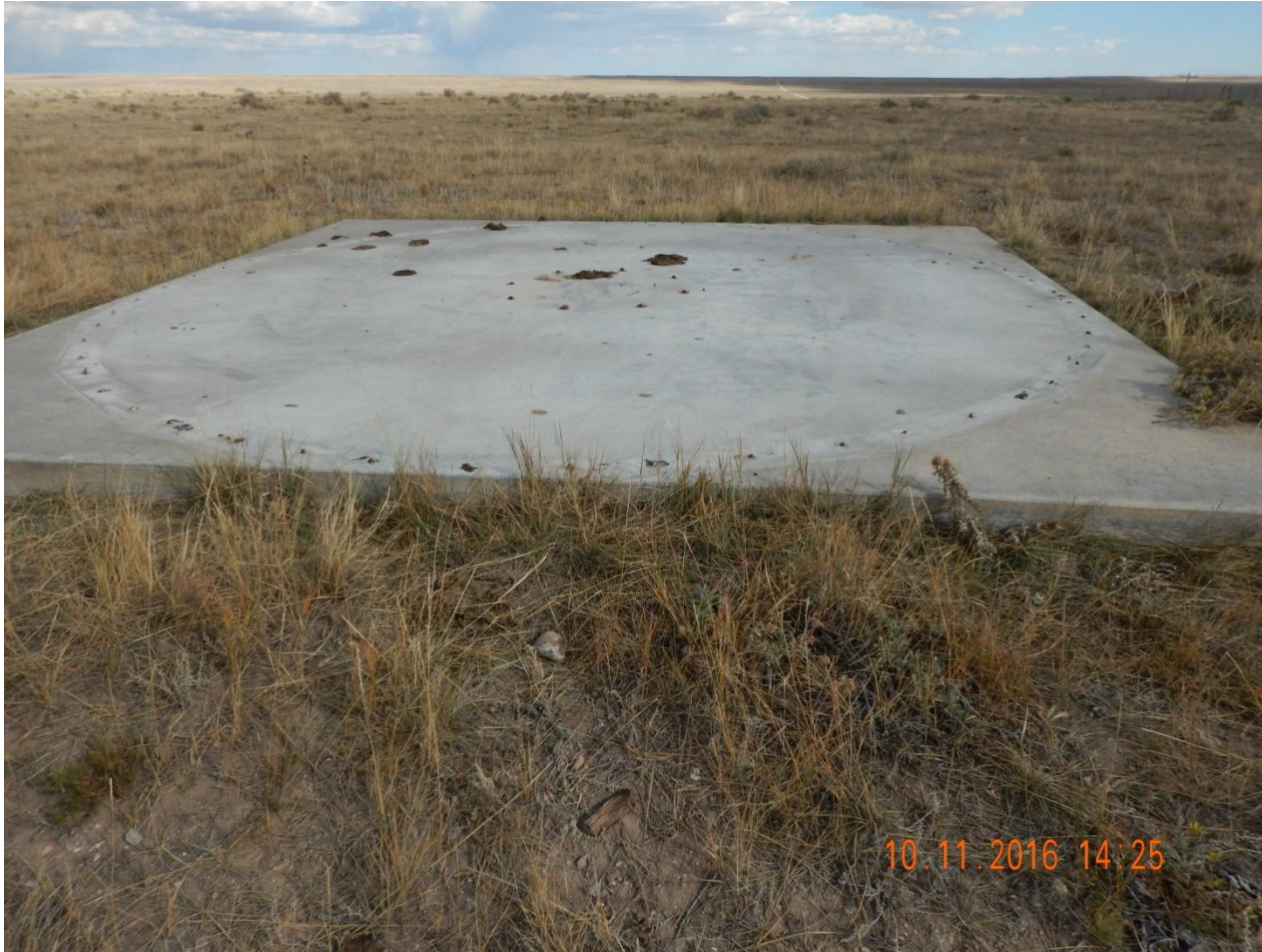
Photo 7. Photo taken from tank battery location. Concrete slab needs to be removed per Rule 1004.
