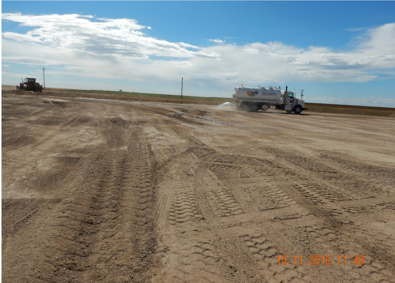
Photo 4. Photo taken from center of location, facing South. Water truck on location to control fugitive dust from operations.
