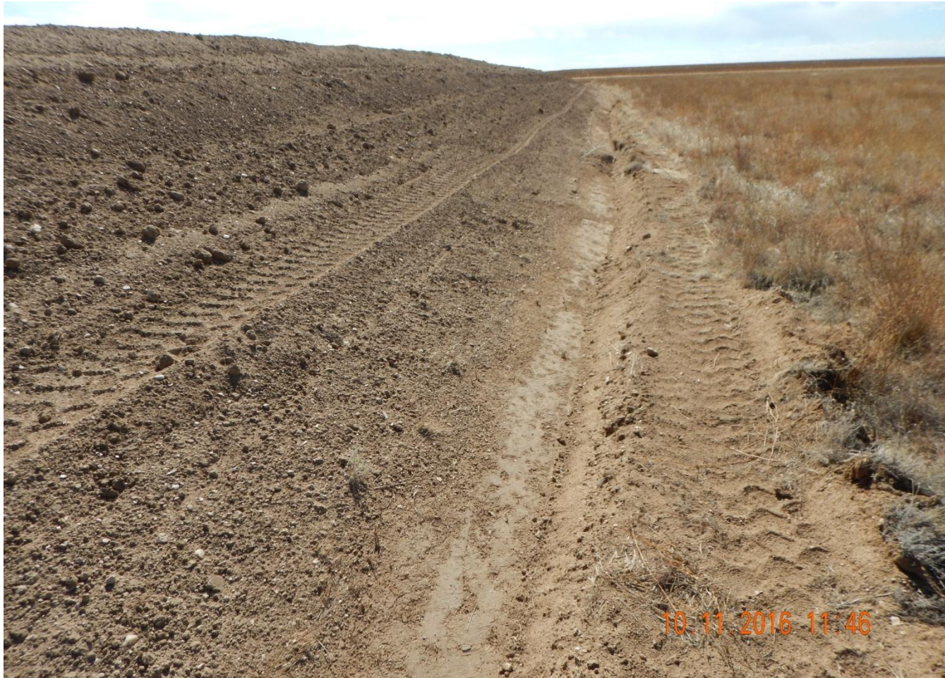
Photo 3. Photo taken from the western soil pile, facing South. Ditch and berm constructed around outer perimeter of subsoil pile. Contractor will re-cut ditch to a wider and deeper depth.
