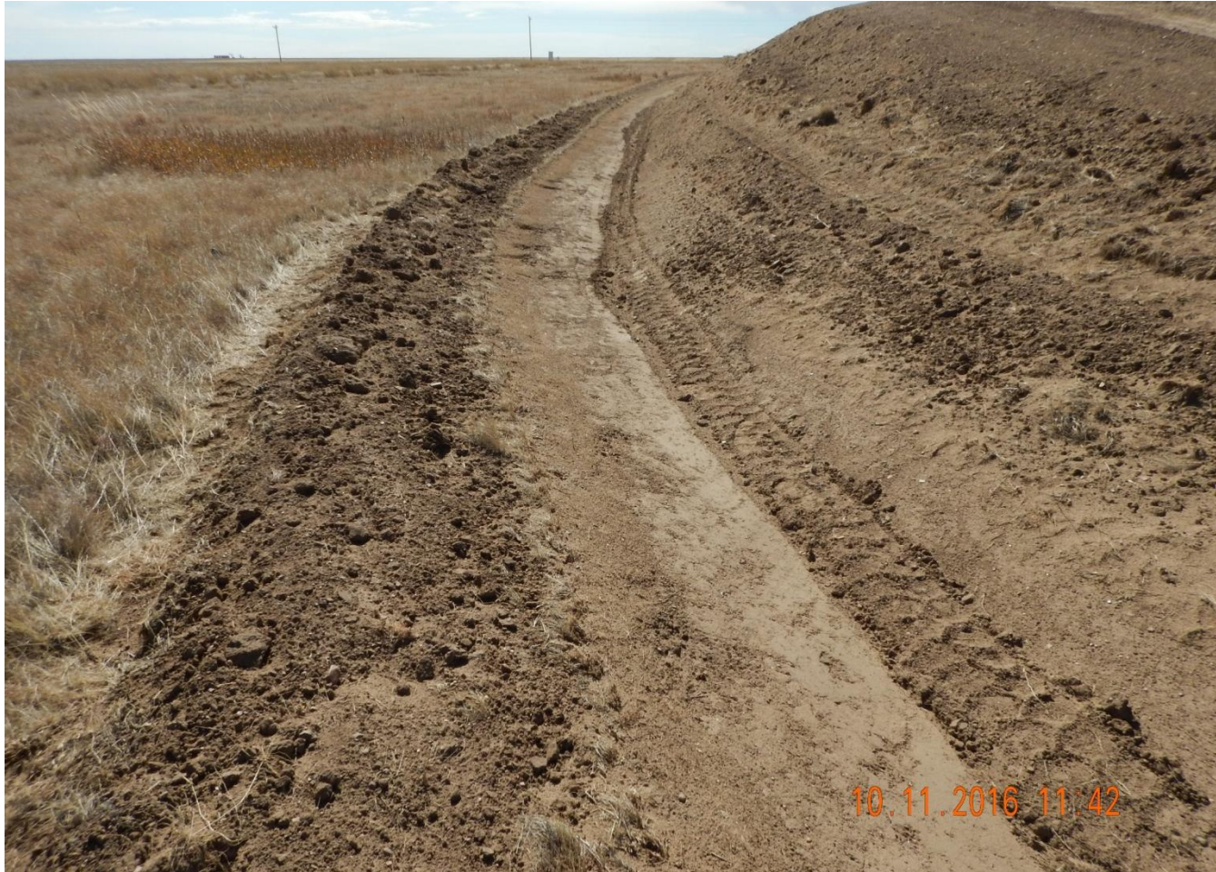
Photo 2. Photo taken from the eastern topsoil pile, facing South. Ditch and berm constructed around outer perimeter of topsoil pile.
