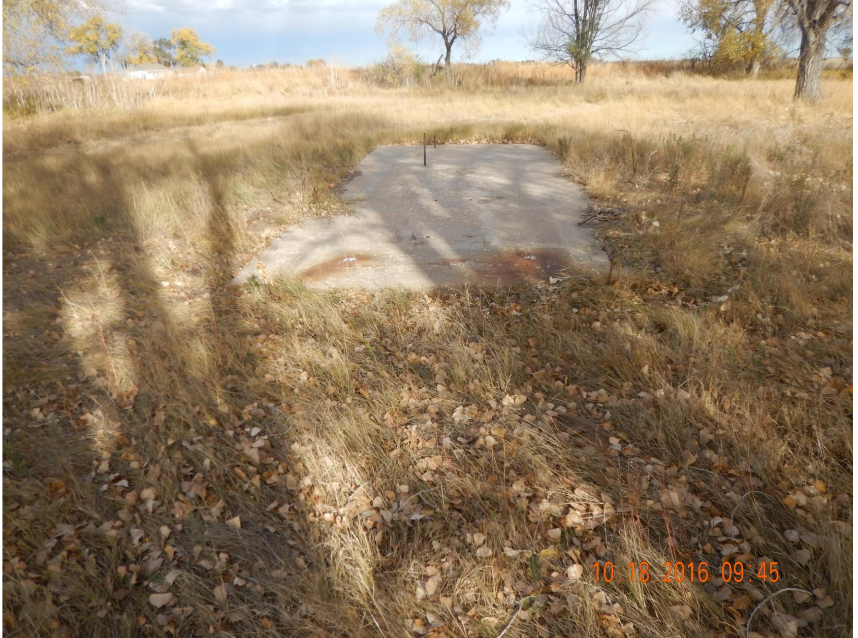
Figure 2: Photo taken from the location, facing north. Photo shows concrete pump base has not been removed.
