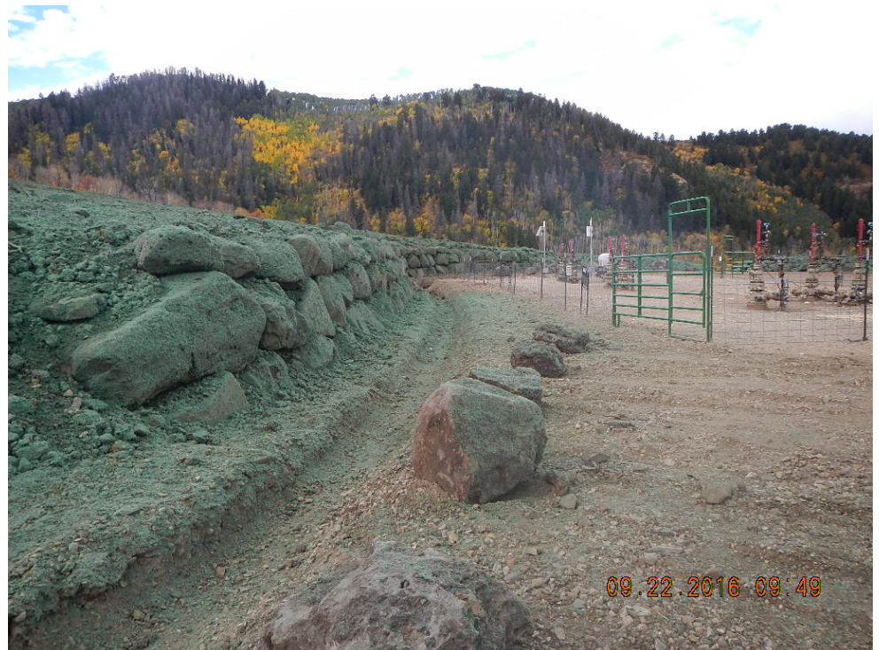
Rock wall and drainage on cut slope side of wellheads.
