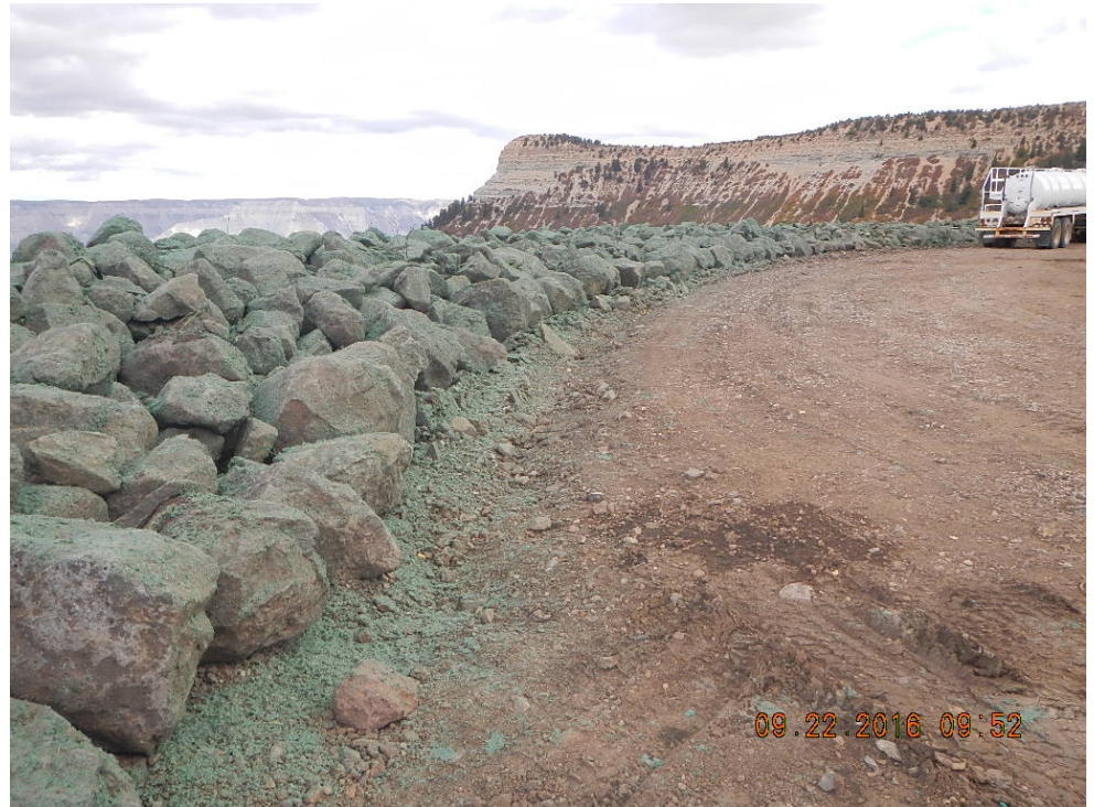
Berm on fill side of location
