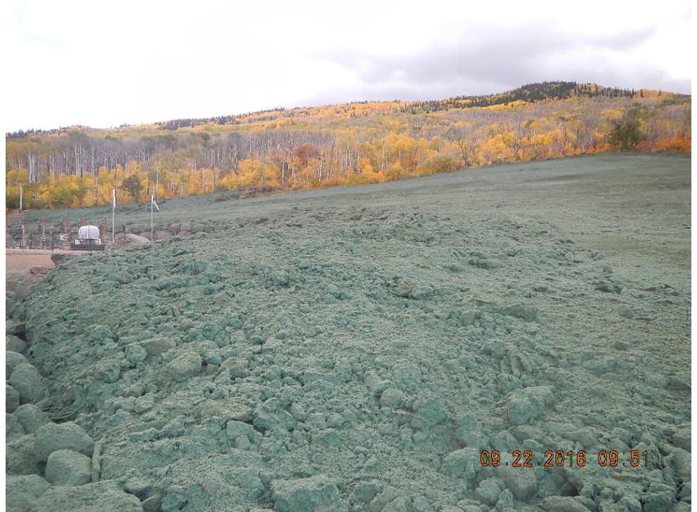
Reconstructed slope where subsidence was
