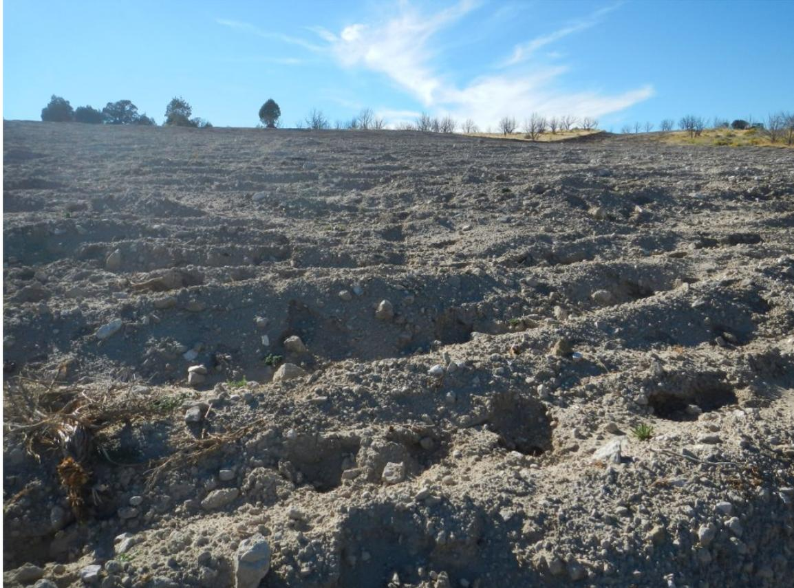
**Photo#2:** View Up Slope to NW; Slope Roughening has been effective.
