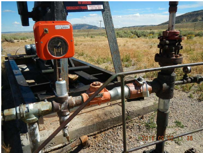
Valve locked out.
