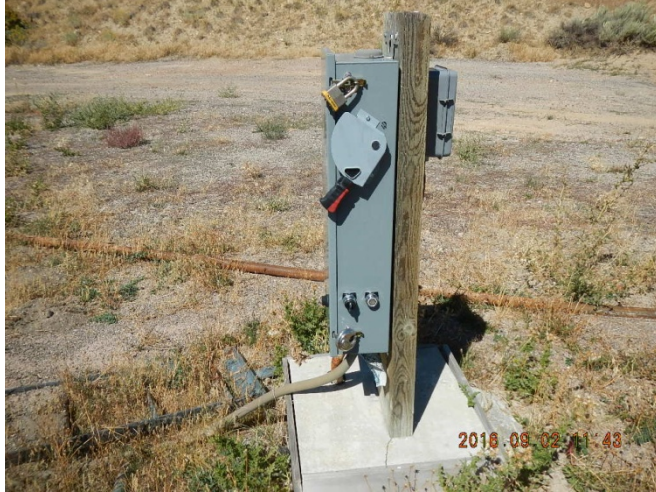
Electrical locked out.
