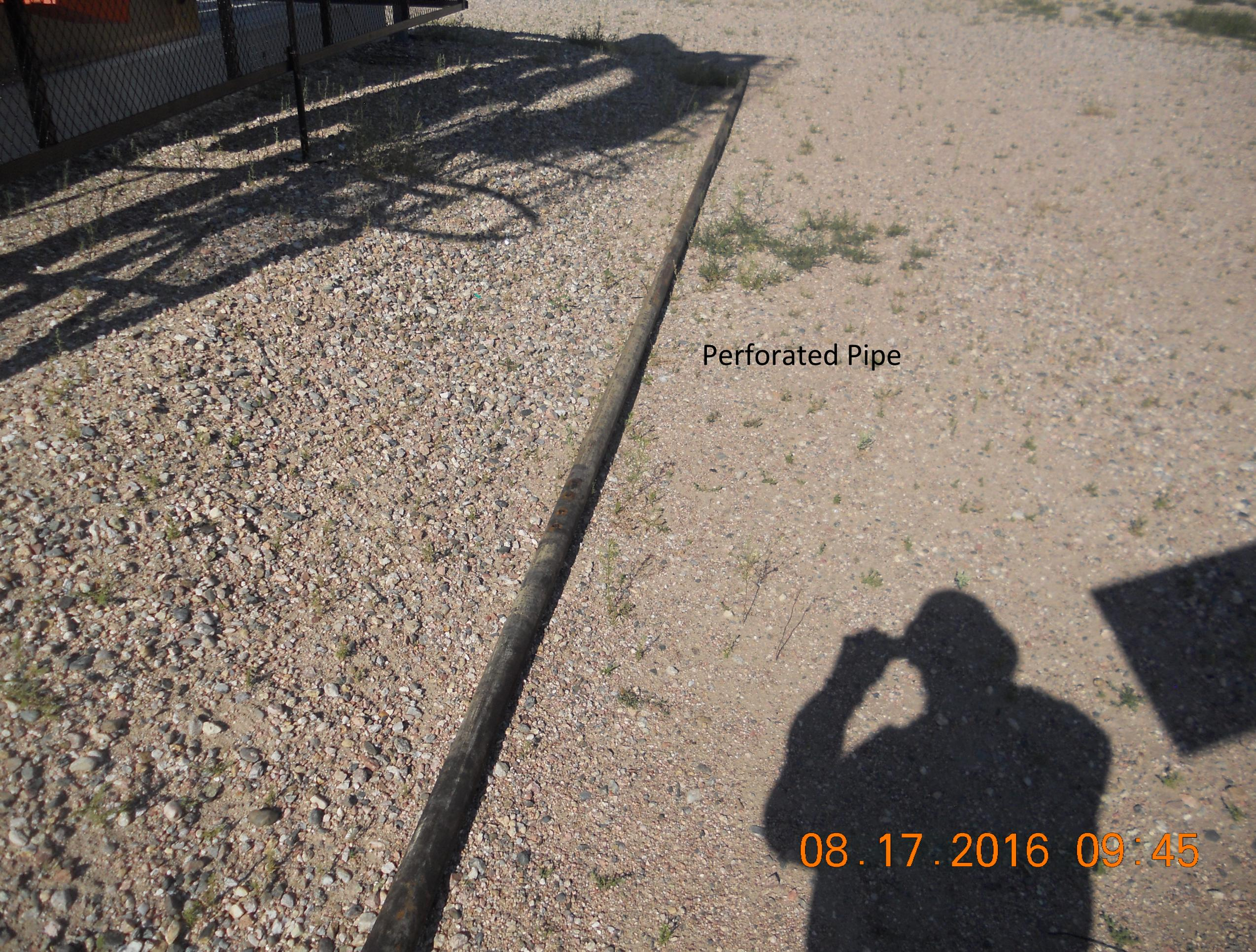
A long, dark, perforated pipe lies horizontally across the middle of the frame. The pipe is set against a background of light-colored gravel and sparse green vegetation. To the left, a chain-link fence runs parallel to the pipe. The scene is brightly lit, casting distinct shadows. The text 'Perforated Pipe' is overlaid in black on the right side of the pipe.
